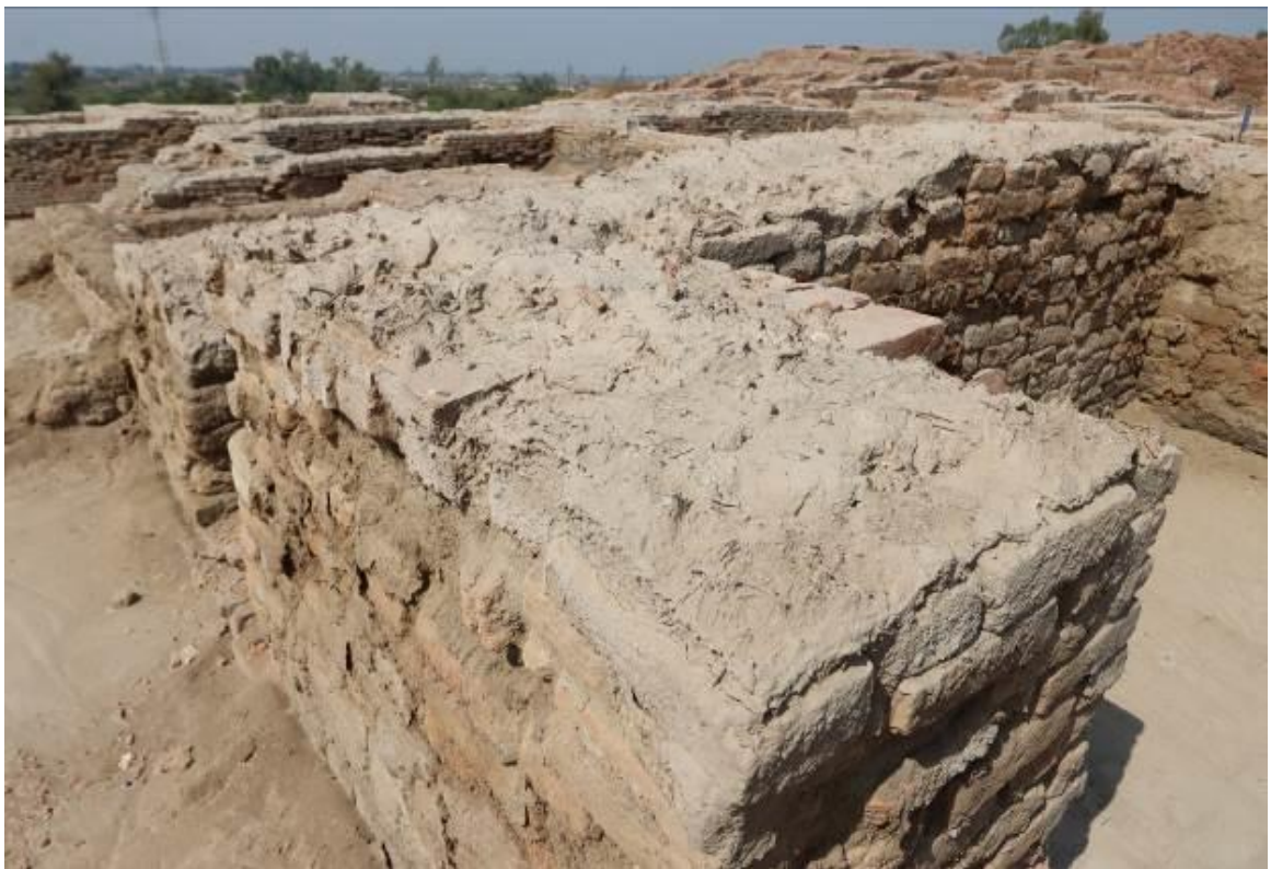
Same type of soil applied on wall capping at SD Area
