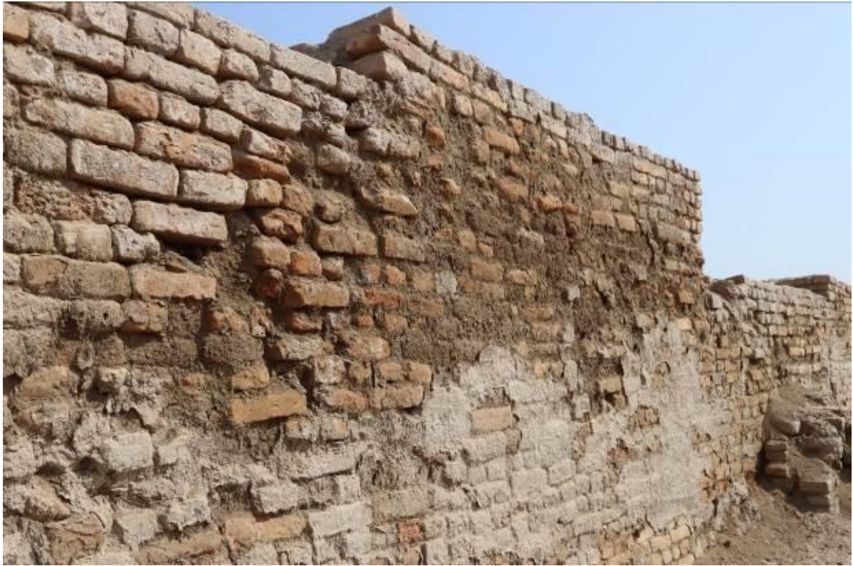
Traces of high humidity on retaining wall, SD area
