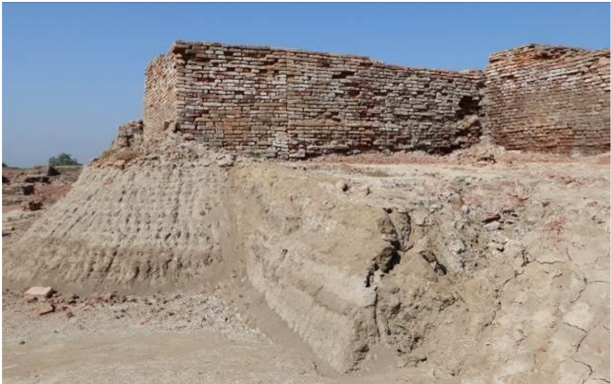
Pushta protection affected by water infiltration HR area
