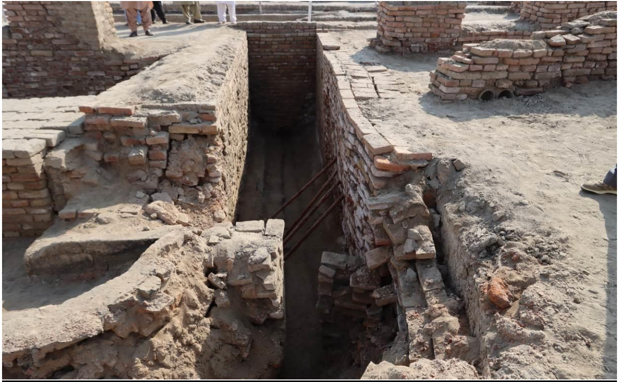
Instability of retaining wall at the southern side of canal from bath in SD area.
