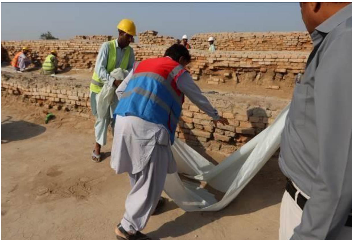
Removal of salty mud slurry, SD Area, using geotextile to collect and transport dust away from the site
