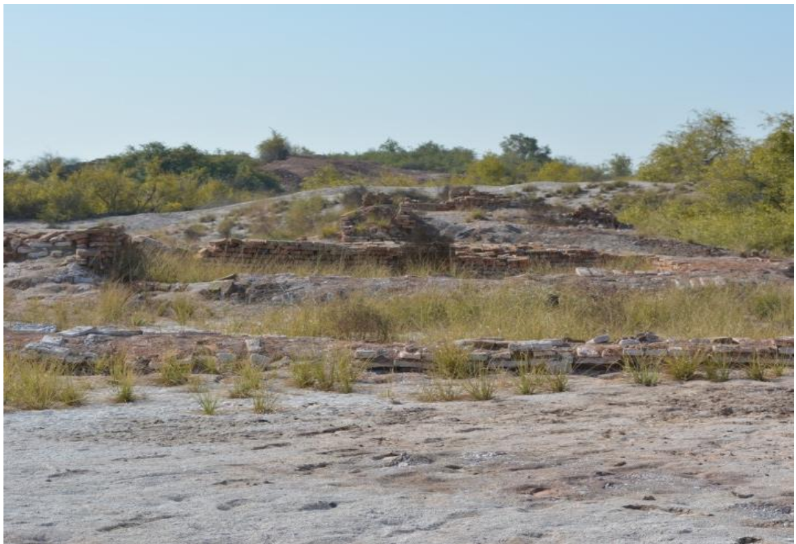
Mud brick capping and resetting of loose brick walls. Resetting of loose bricks by relaying the loose and decayed courses of the brick walls exactly similar to the original
