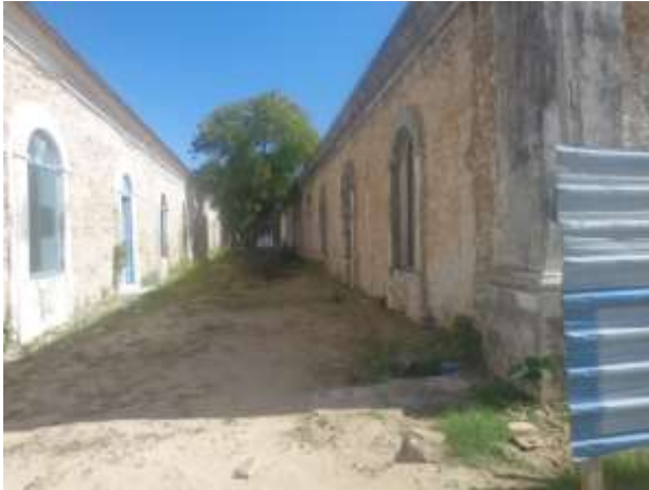
Four (04) compartments in the process of recovery (GACIM 2022)
