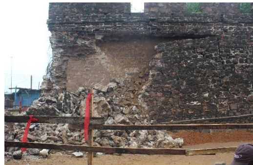
Crumbled section of fort wall
