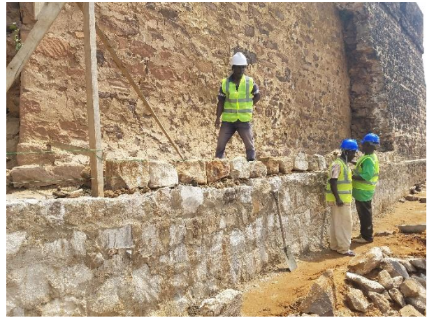
Masons laying stones wall above the plinth
