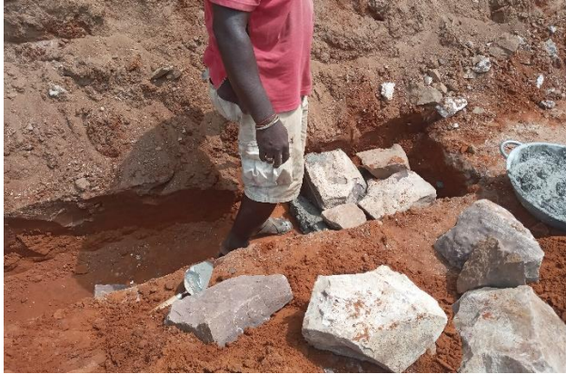
Foundation receiving first set of boulders
