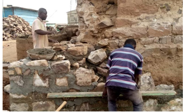
Ensuring straightness of wall (plinth) with a rod
