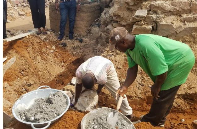
Foundation receiving first set of boulders
