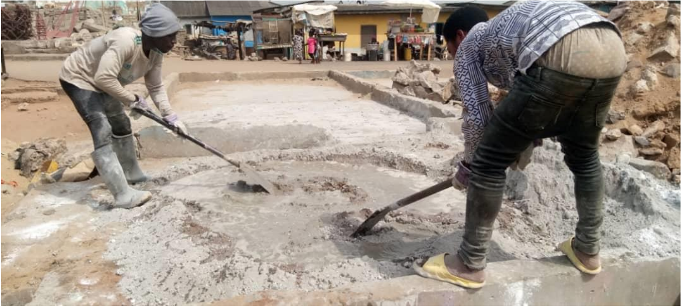
Mixing of mortar by labourers
