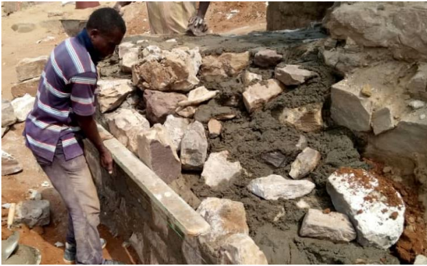
Ensuring straightness of wall (plinth) with a rod
