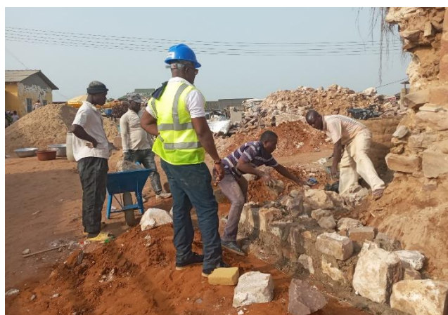
Masons laying stones of plinth above ground level
