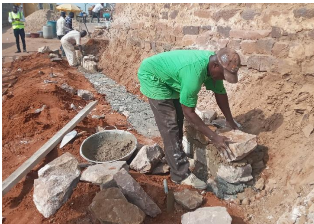
Masons laying stones of plinth above ground level
