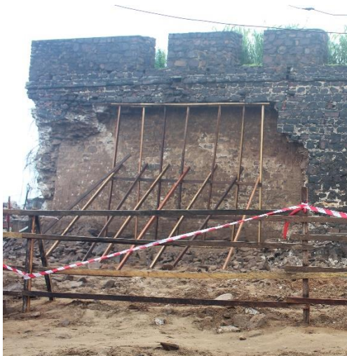
Hanging portion of crumbled wall propped with timber
