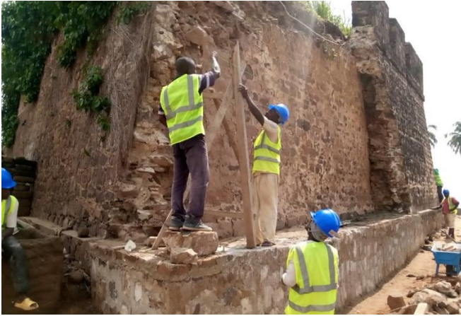
Masons creating a temporary structure to guide the reconstruction of the sloppy wall.
