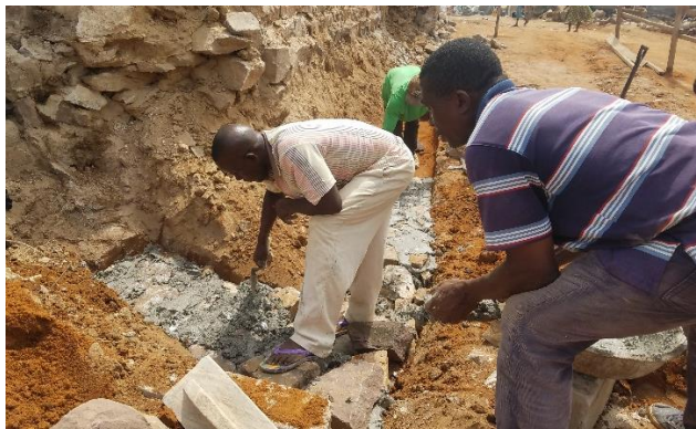
Foundation boulders laid almost to existing ground level
