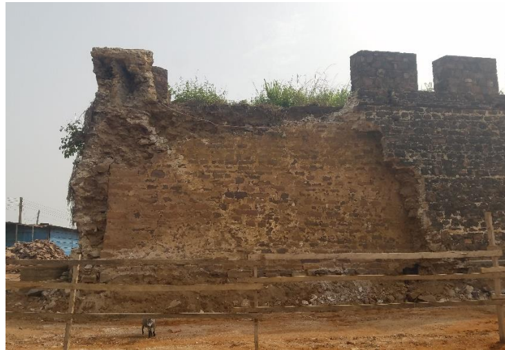
Crumbled section of fort after hanging portion has also fallen off.
