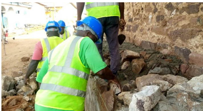
Masons laying last set of stones for the plinth
