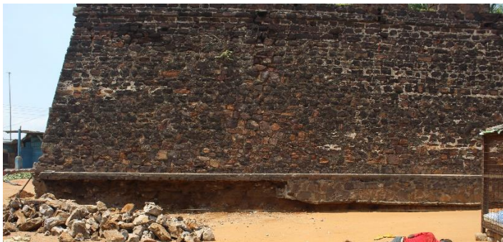
Wall during preparatory works to consolidate plinth/apron – Pre collapse.
