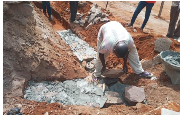
Foundation boulders laid almost to existing ground level
