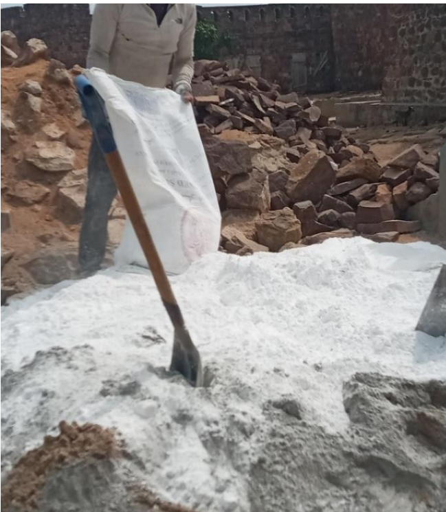
mixing of mortar by labourers
