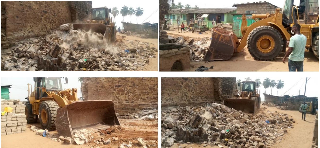
Payloader from Amandi helping to clear and heap debris on site.
