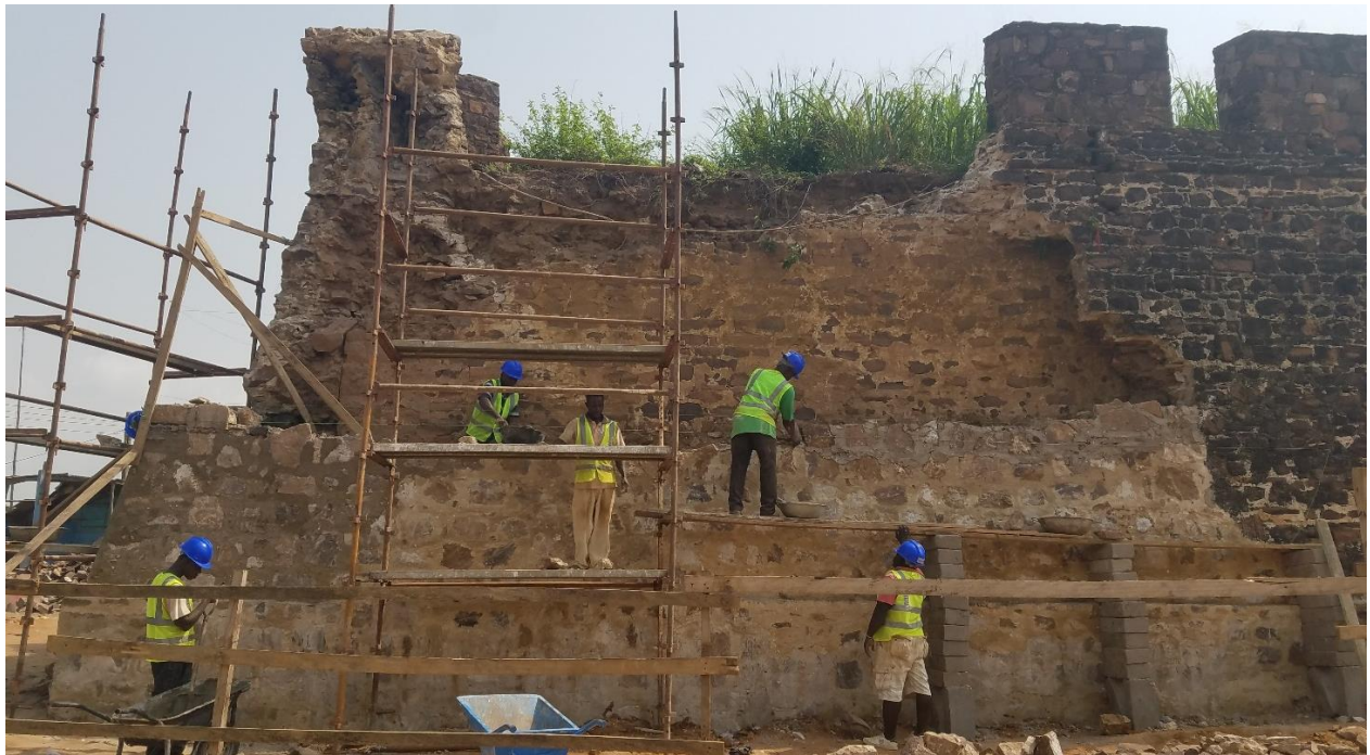
Scaffolds were employed as height of wall increases
