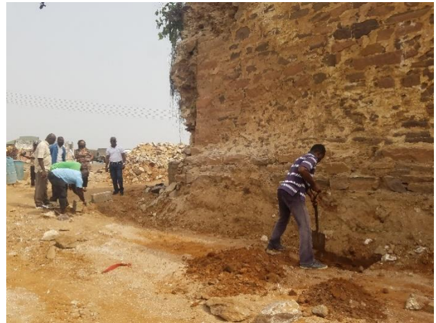
Masons excavating foundation trenches
