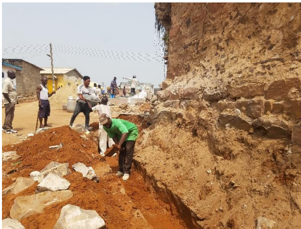
Masons excavating foundation trenches
