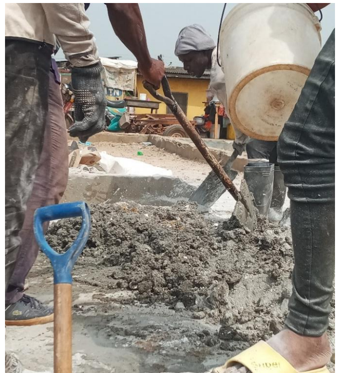
mixing of mortar by labourers
