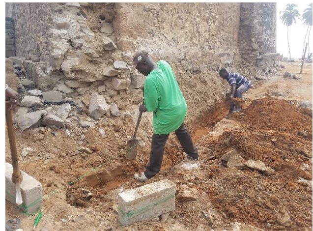
Masons excavating foundation trenches
