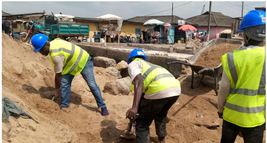
Labourers loading sand into wheelbarrow for batching and mixing
