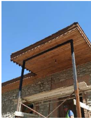
Reinforcement inside of columns
