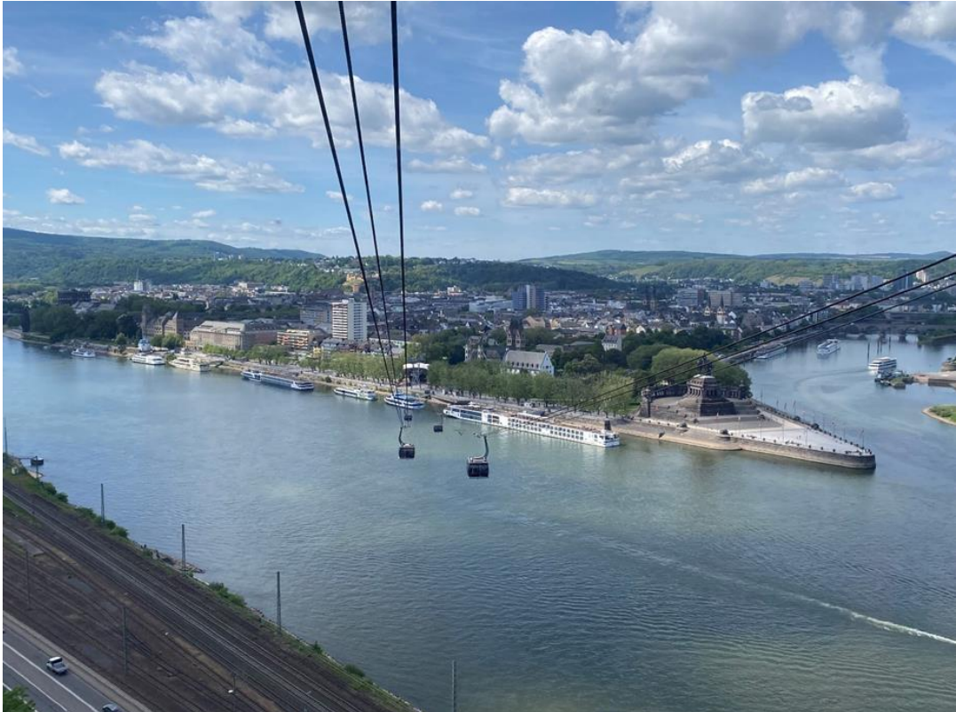
The area of the 'valley station' for the cable car in Koblenz (photo: Réka Viragos)
