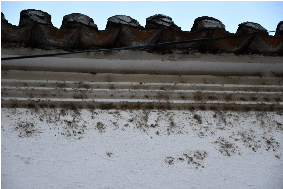
Berat: details of common fungal overgrowth visible on the façades. © K.Piotrowska, 2021
