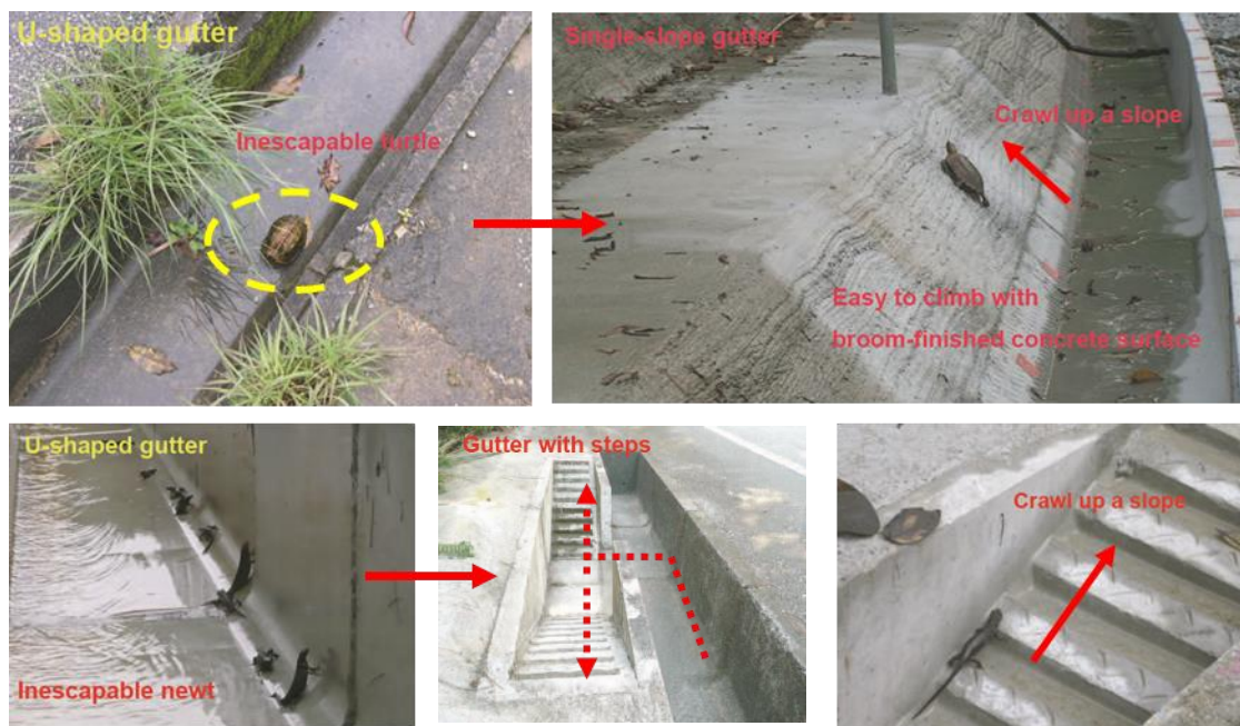
Figure 22: Improvements to single-slope gutter and gutter with steps (Maintenance and Management Section, Okinawa Prefecture Hokubu Regional Public Works Office, 2010)
