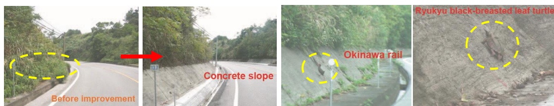
Figure 21: Concrete slopes with roughened surfaces. Okinawa rails and Ryukyu black-breasted leaf turtles have been confirmed climbing up the improved slopes. (Maintenance and Management Section, Okinawa Prefecture Hokubu Regional Public Works Office, 2010)
