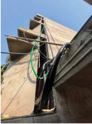
Image 21: Electric Cable on the Facade
