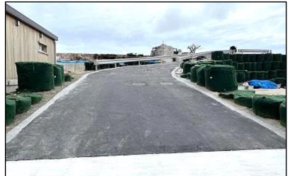
Temporary road for construction (north ramp)
