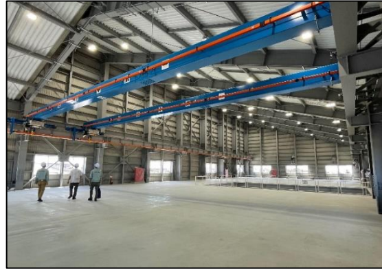
Temporary lumber storage and wood-processing plant (interior)
