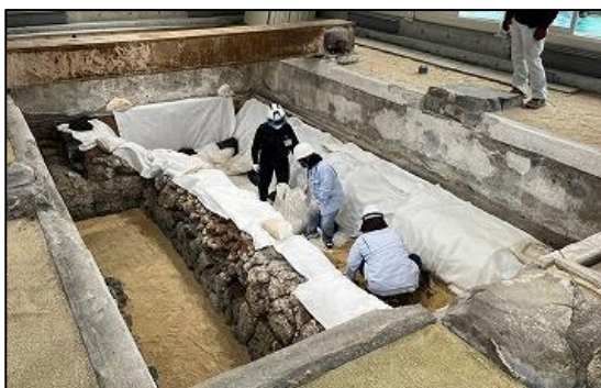
Protection by sand capping on remains for preparation of the rebuilding work of state hall
