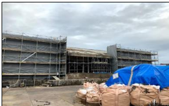
Hokuden (northern hall) (Before dismantling)
