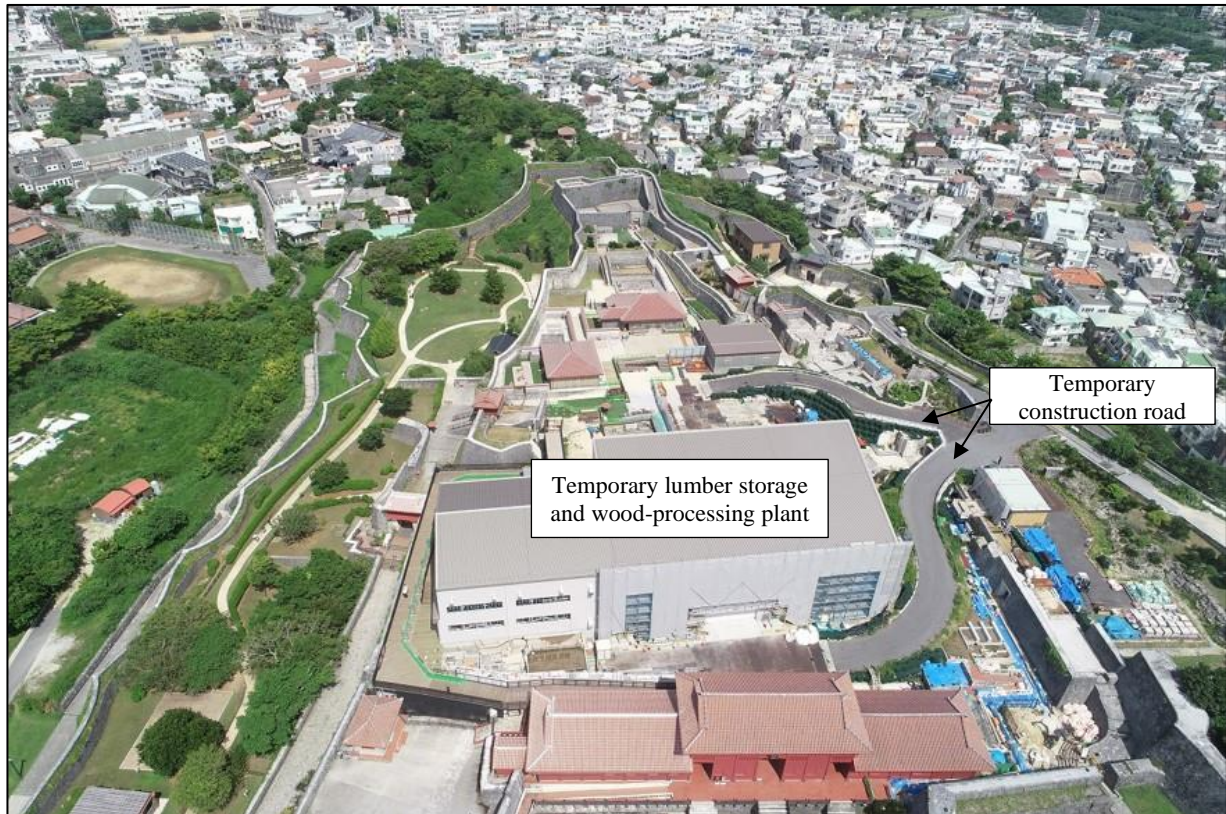
Up-to-date view of Shuri-jô site (August 2022)
