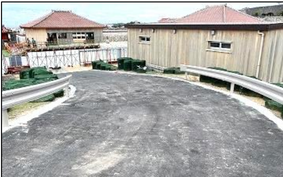
Temporary road for construction (south ramp)
