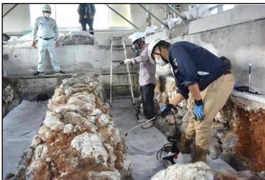
Resin reinforcement
