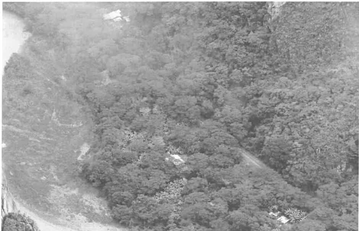
Photo 4.5. Railway tracks to the Amazonian Access at the valley of the río Vilcanota seen from the Wayna Picchu. Photo 4.6. Incipient developments along the railway tracks to the Amazonian Access.
