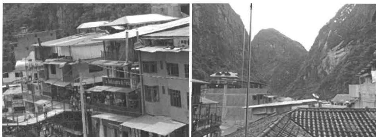
Photo 4.9: Buildings heights and roofs
