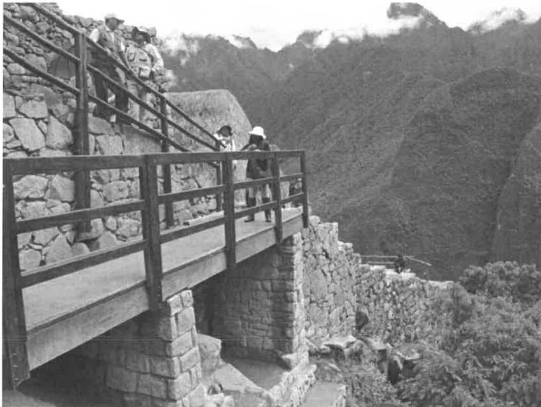
Photo 4.15. The entrance (left) and the new exit ramp (right).
