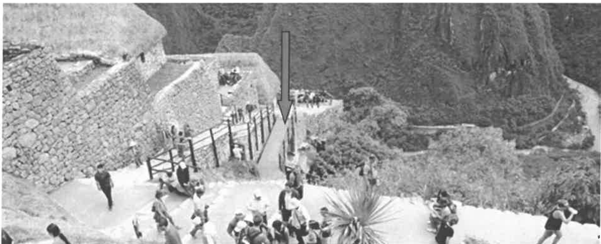
Photo 4.13. The entrance / exit area of the Llaqta with the new exit ramp (marked with a red arrow).
