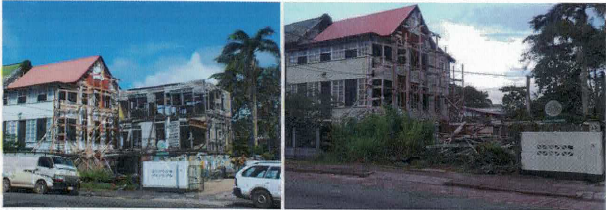
Demolition of Grote Combéweg 13
