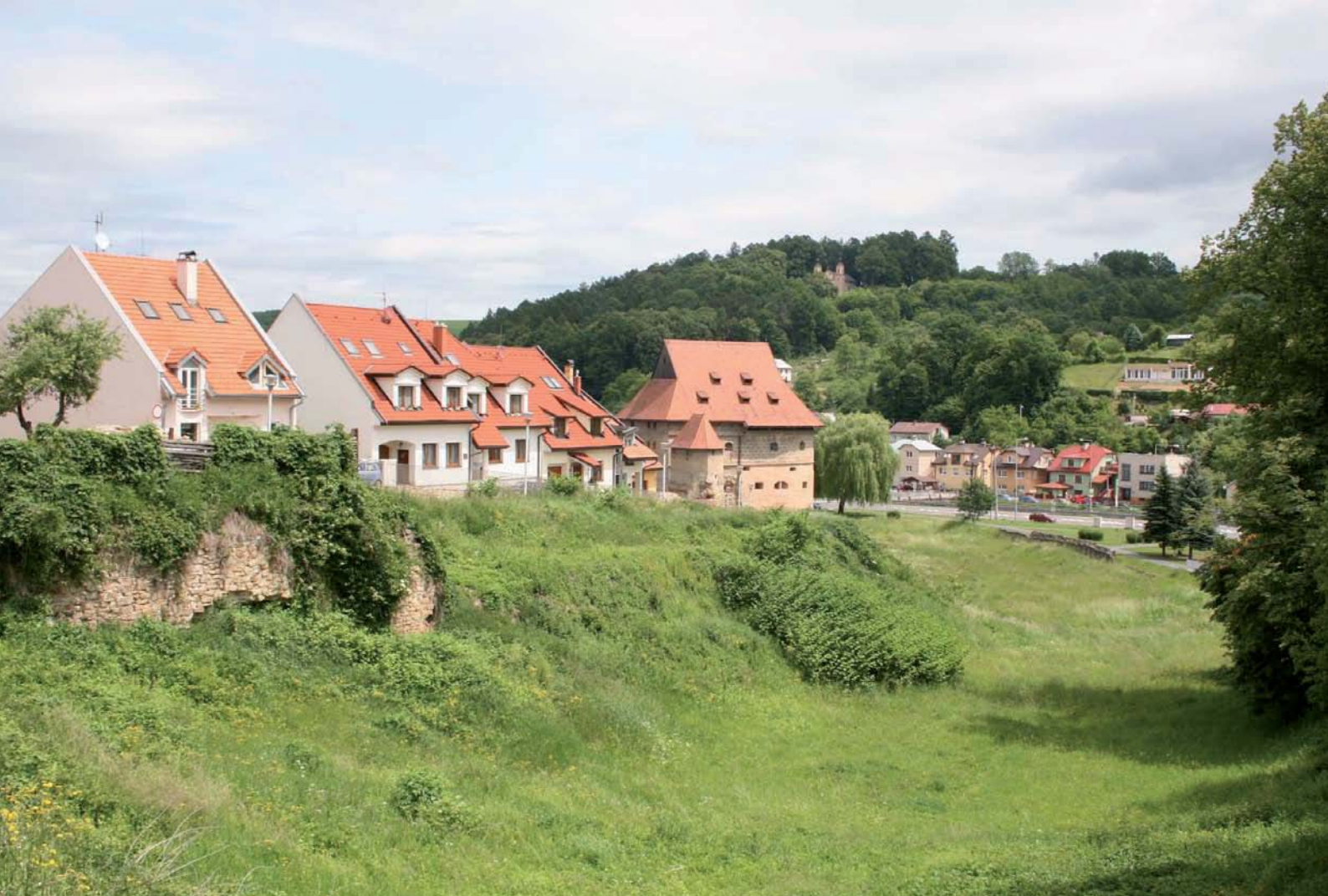
Built-up area along the southern part of the fortification with the view of Hrubá bašta (Thick Bastion) and the Calvary
