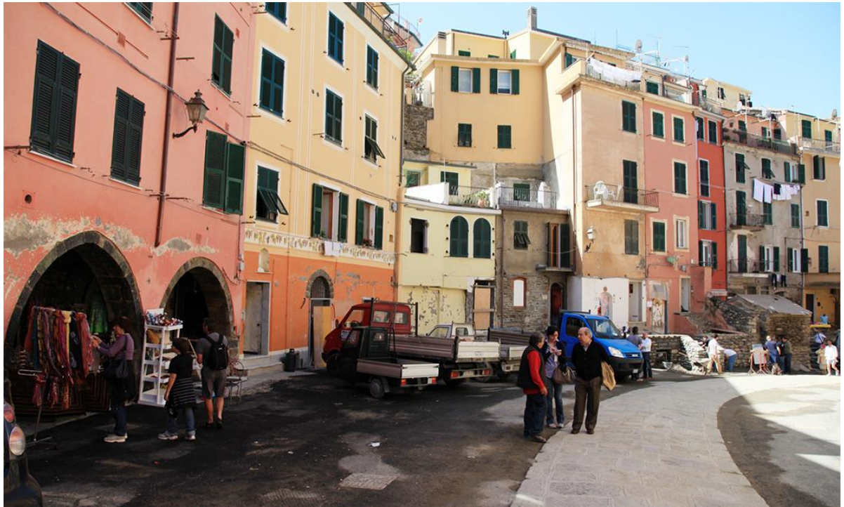
Figure 22. Via Roma before the intervention
