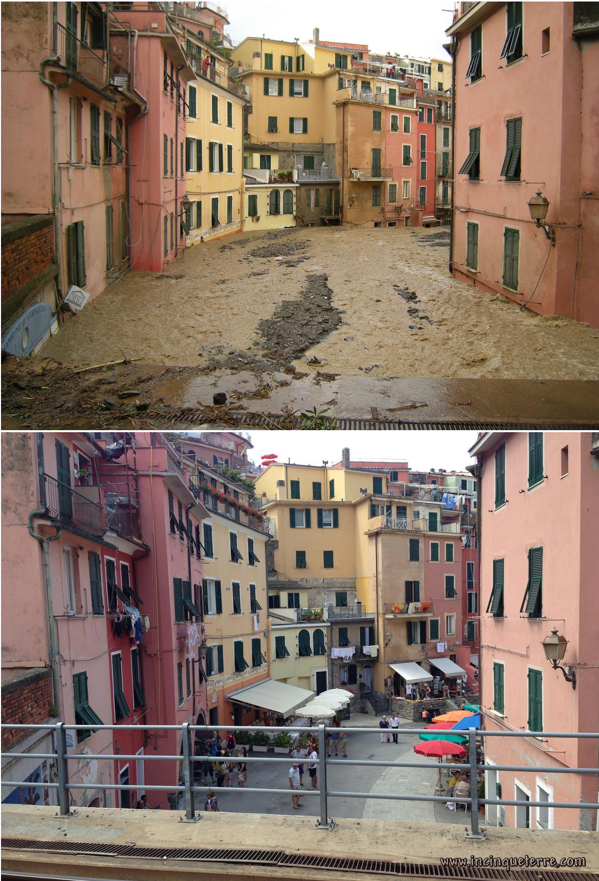
Figure 2. View of Via Roma after the flood and after the cleaning (source: www.incinqueterre.com )
