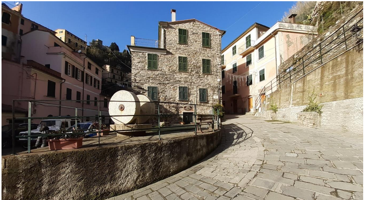
Figure 7. Use of Carniglia sandstone for flooring
