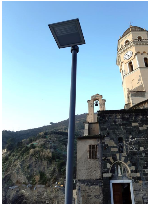
Figure 32. Lighting in Piazza Marconi after the restoration
