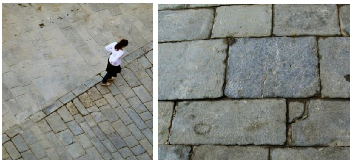
Figure 27. Flooring before the intervention
