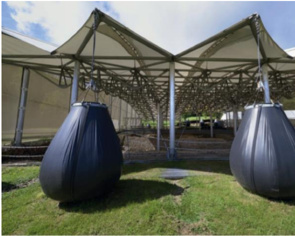
Figure 198: Stretched velum on an archeological site with ballast (without anchorage) – BIBRACTE (France)
