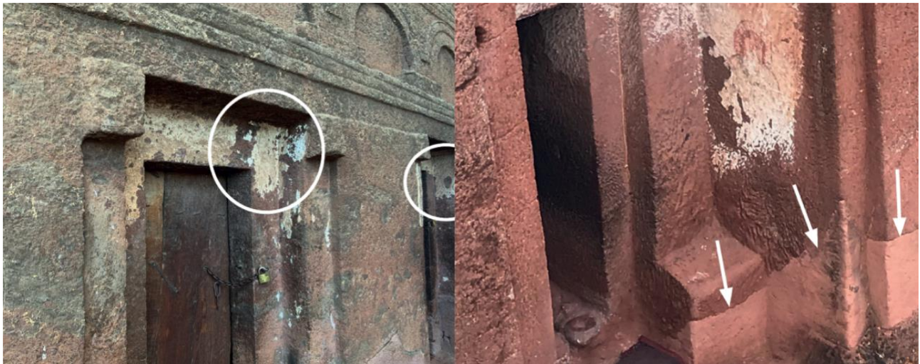
Figure 126: Biete Maskal – South entrances Figure 127: Biete Gabriel Raphael – Contrast of light-coloured mortar patching on the basement
