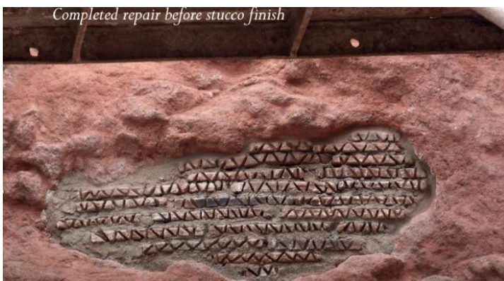
Figure 115: Filling of gaps with mortar-filled rubble (before finishing plaster) Stephen BATTLE June 2016 World Monuments Fund: « Preservation at the Rock Hewn Churches of Lalibela, Ethiopia » (S- LMAQM-12-GR-022-A001)
