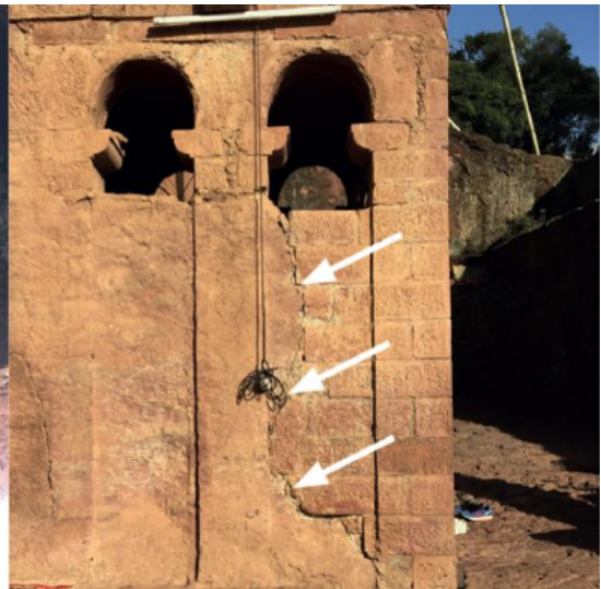
Figure 124: South porch side elevation of Biete Mariam – Dressed stone cladding restored following collapse
