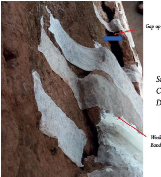
Figure 113: South Façade Biete Maskal – Textured plaster finishing on repairs
