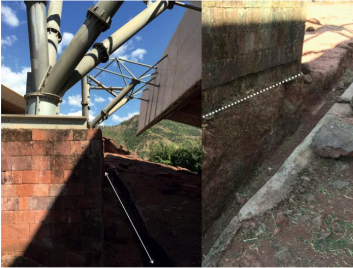
Figure 142: Biete Abba Libanos – Erosion of the foundation at the foot of the shelter
