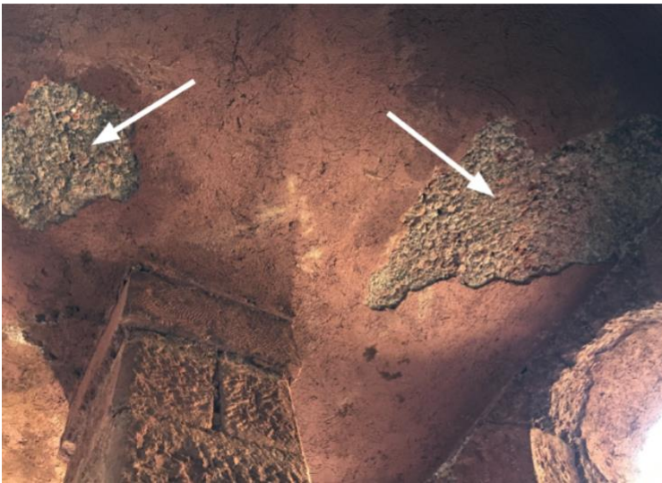
Figure 125: Biete Mariam – desquamation of the plaster under the ceilings of the north porch
