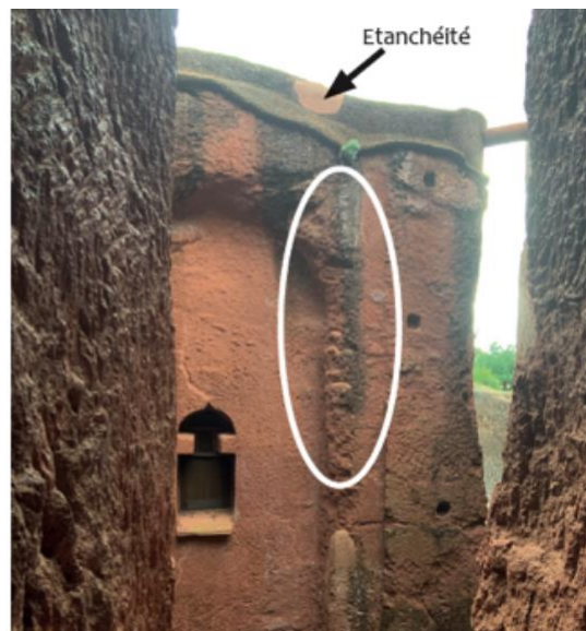
Erosion of façade cladding
