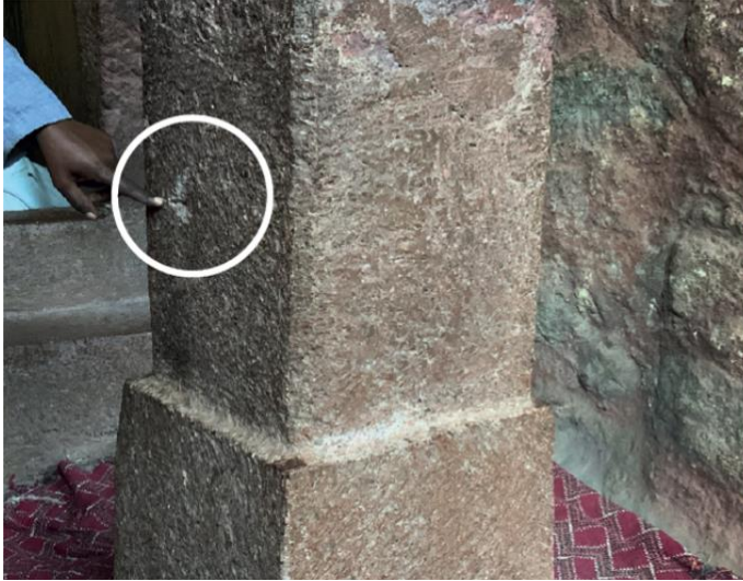
Figure 117: North Porch Biete Mariam – Pillar rebuilt with mortar
