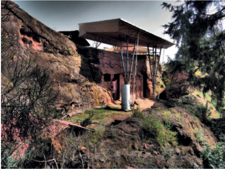
Figure 204: Support of panels for plateau shelters
