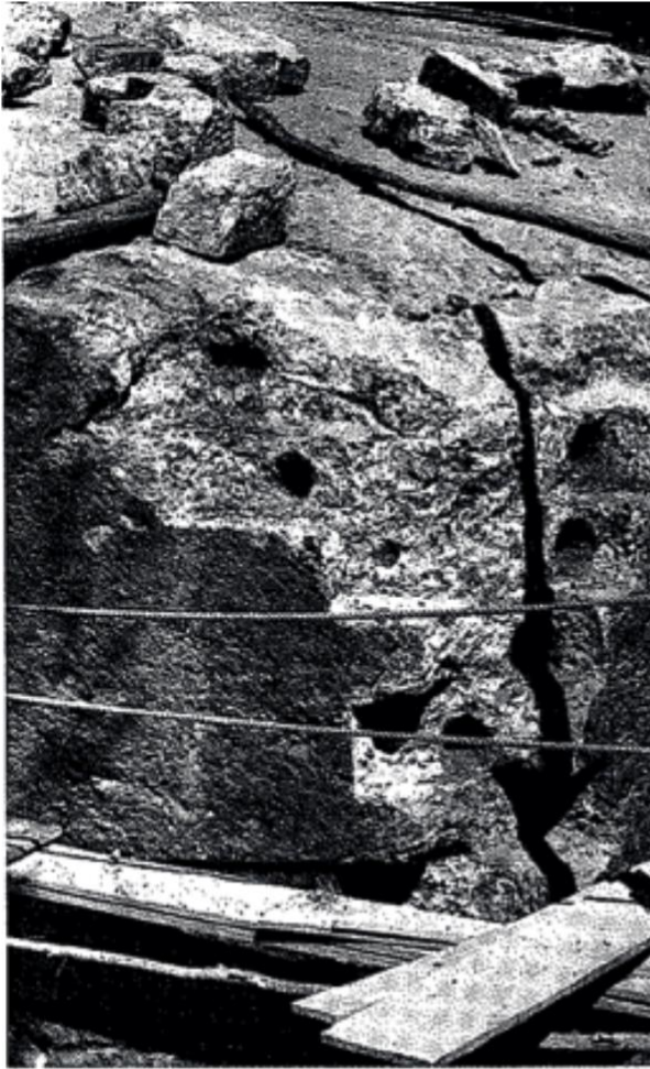
Same corner after removal of incongruous additions but before restoration to monolithic form and appearance.
