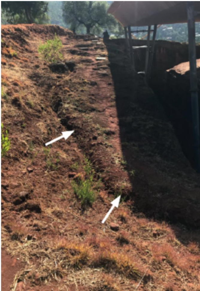
Figure 89: Surroundings of Biete Amanuel – Surface Stream Collection Channel
