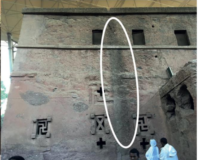
Figure 105: North façade of Biete Mariam – Vertical guttering under the gargoyle
