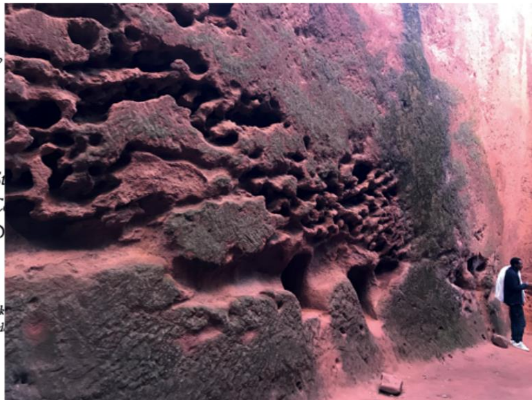
Figure 114: Biete Abba Libanos – Alveolisation of the courtyard walls
