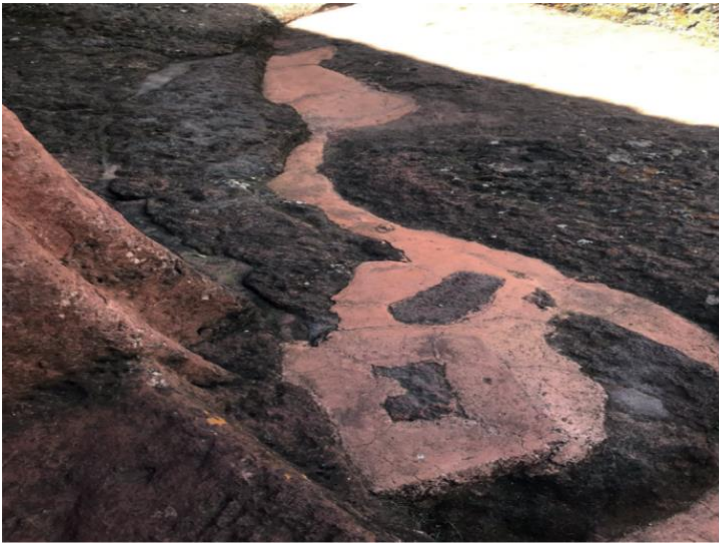
Figure 133: Biete Gabriel Raphael – Crack filling with mortar
