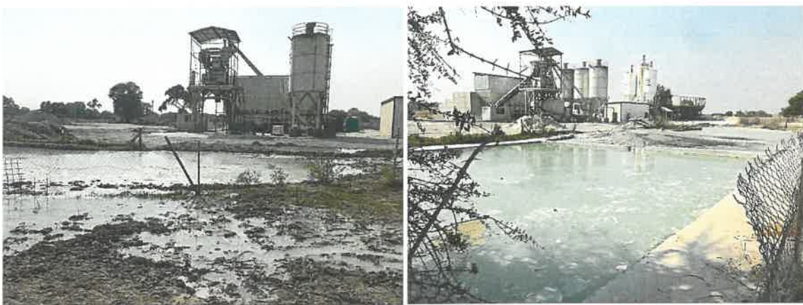
Figure 7. Liquid waste management at Cement-batching Plant
