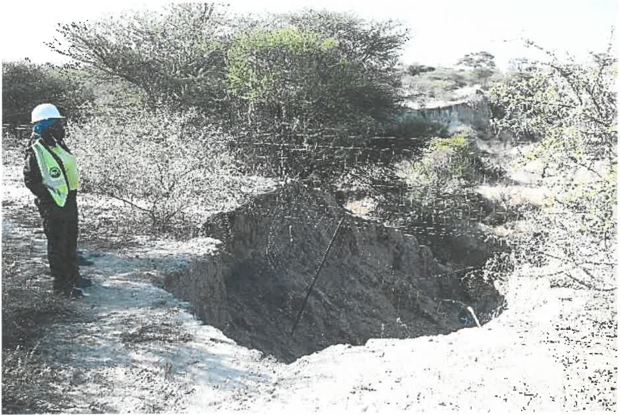
Figure 1. Gully encroaching into fence at Samochima Burrow Pit
