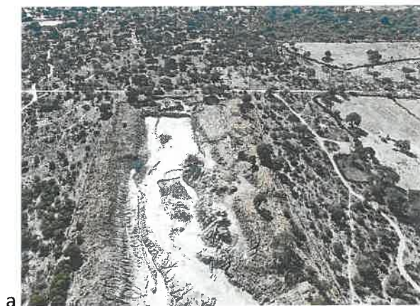
Figure 3 Aerial view of Burrow Pits at Samochima
