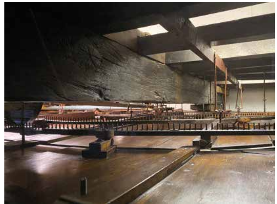
56. 57. The space above the ceiling [mezzanine], housing the combination of pendulum clock and cogwheels, which functions as a gear.
