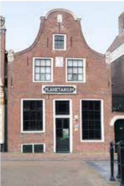
46. The building Eise Eisingastraet 3 is the load-bearing structure for the planetarium instrument.
