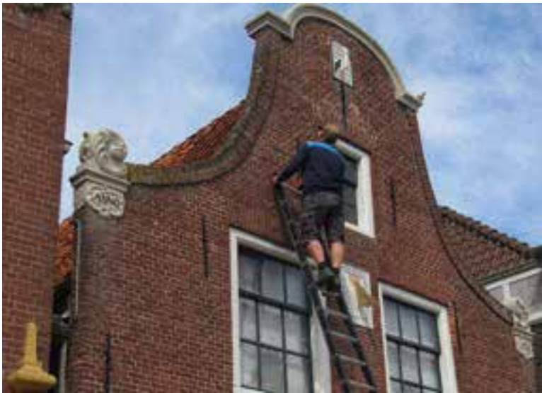
188. Monument Watch Fryslân Foundation.
