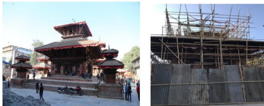
Soon after Earthquake-2015 Restoration in progress-2020
