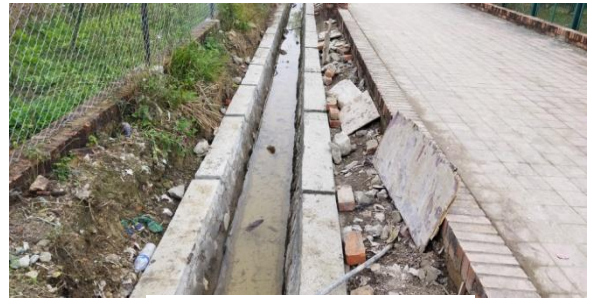
Maintenance work on progress
