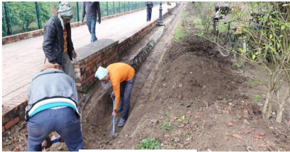
Cleaning old drain
