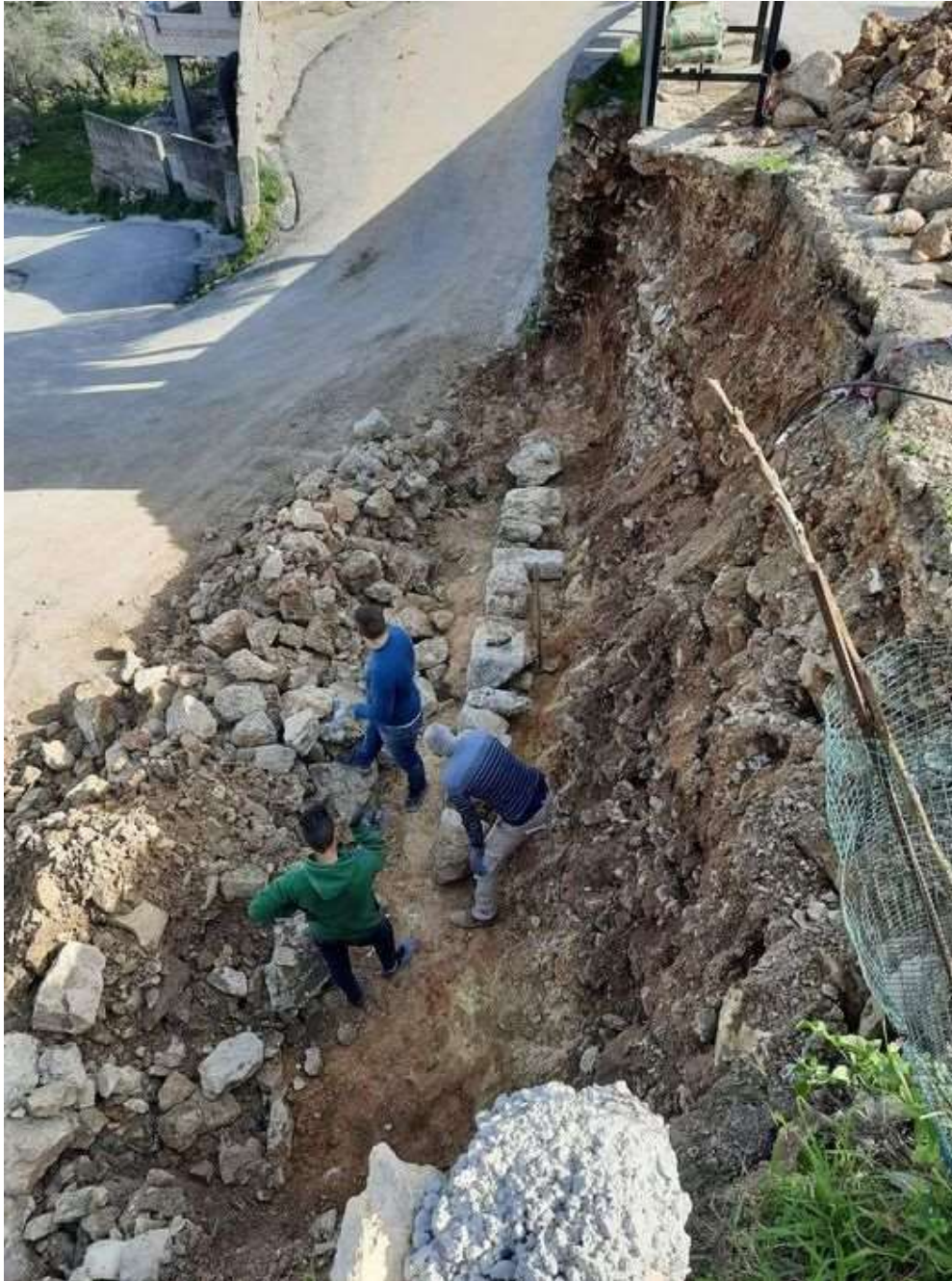
Figure 15:- Rehabilitation of Dry- stone Walls in the WHP.
