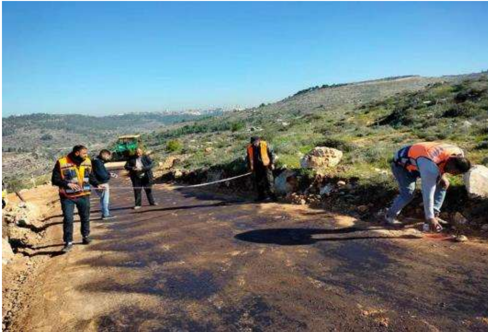
Figure 13:- Rehabilitation of Karm Hadidoun Road
