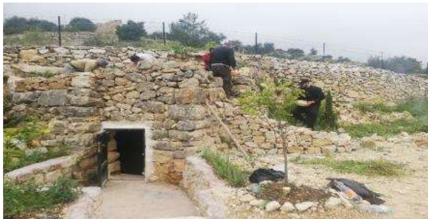
Figure 8:- Renovation Project of Watchtowers in al-Makhrou Area
