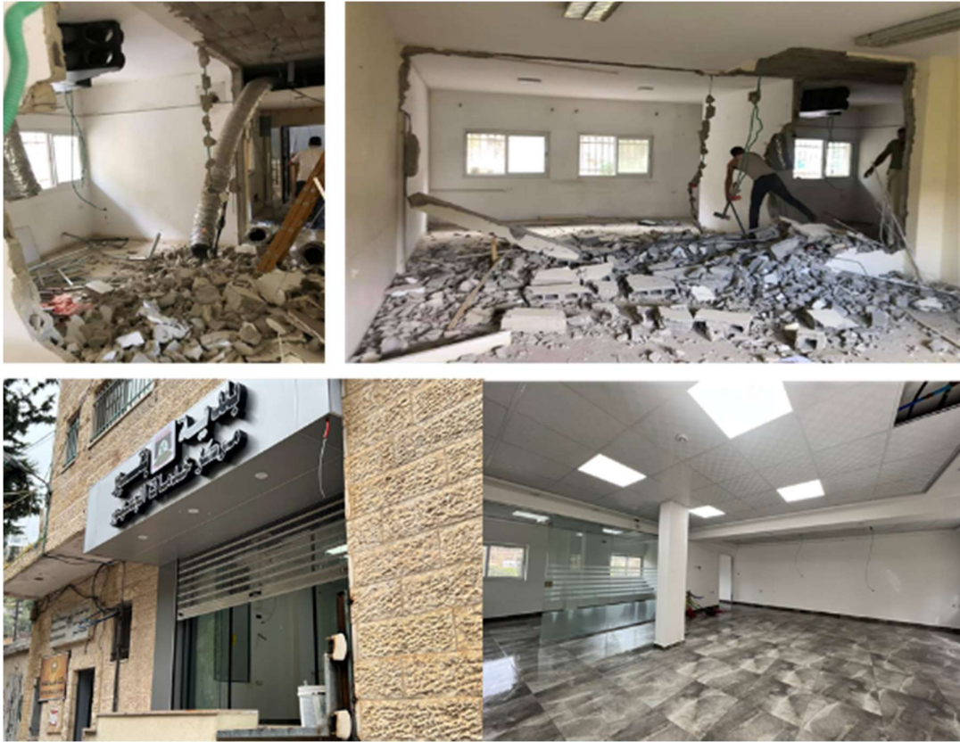
Figure 12:- Rehabilitation of the Public Service Center
