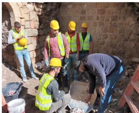
During the training course of conservation of stone façade
