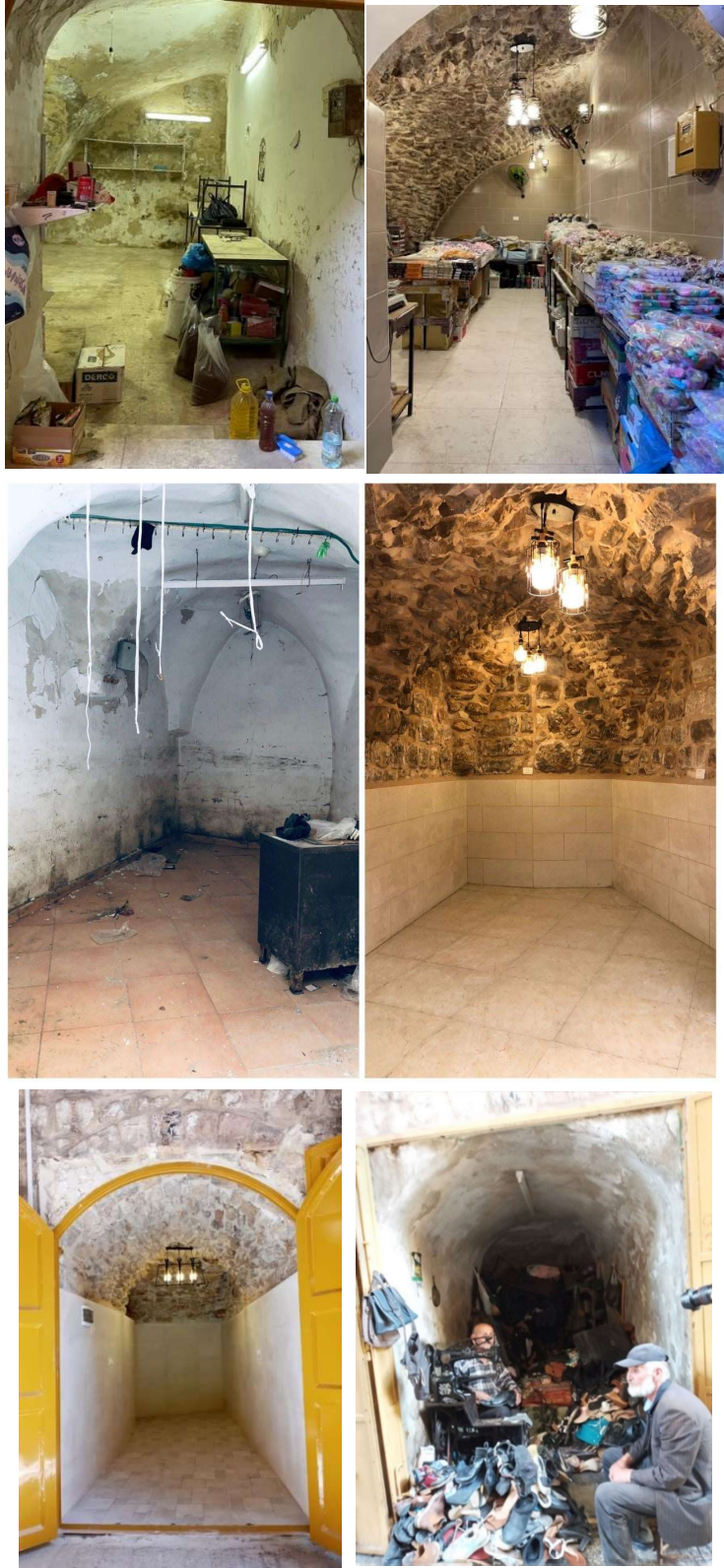
Rehabilitation of commercial stores (before &after)
