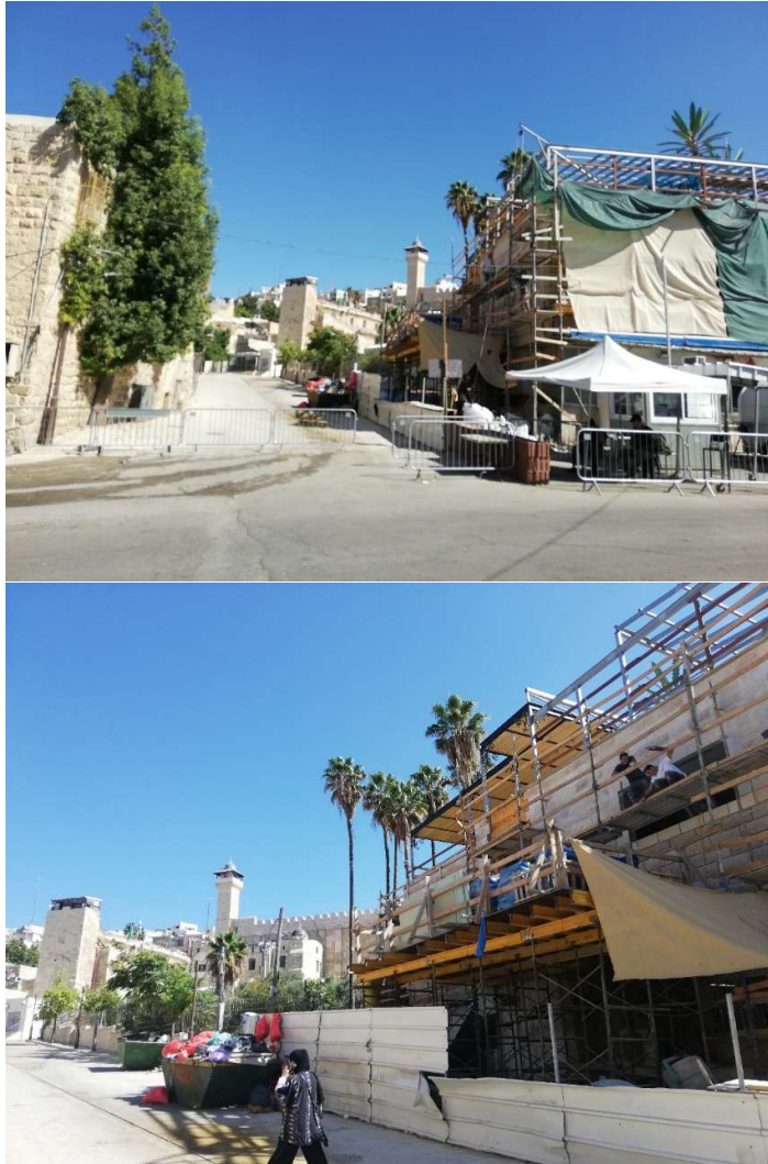
Building new concrete-stone stories in front of the Ibrahimi Mosque
