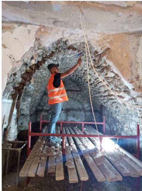
During conservation of commercial stores
