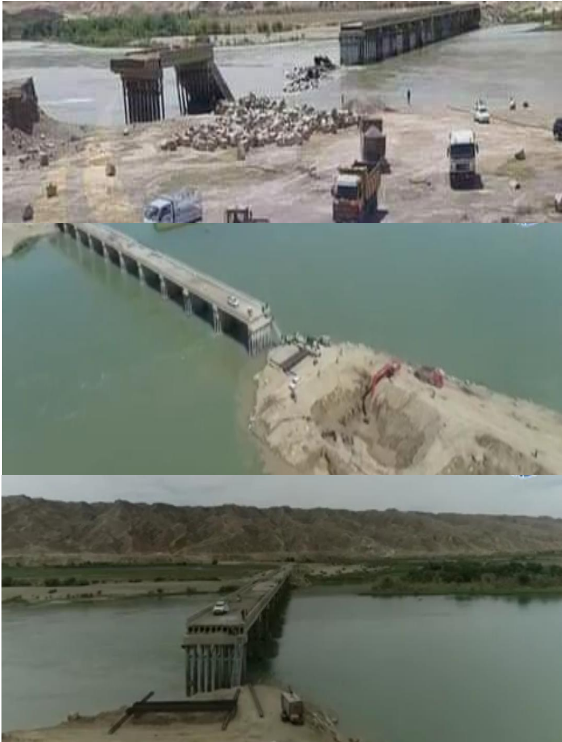
(Figure 1) Ongoing Works in Makhoul Dam (Rehabilitation of the Service Bridge)
