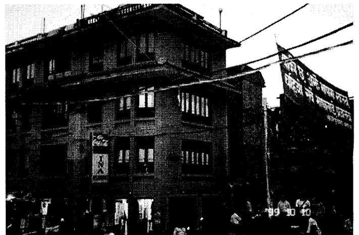
(Below left) The ground floor of a fine traditional building in Patan was replaced in 1998 with a concrete framed ground floor (below right), with modern openings. 4 traditional windows have disappeared.
