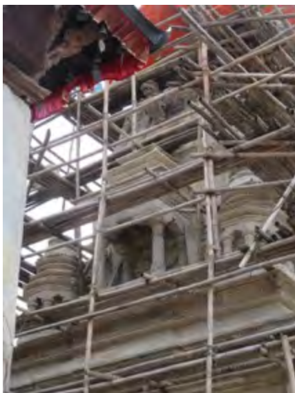
Reconstruction of the Batsala Devi Temple incorporates the original stone and some new stone elements to replace what was destroyed in the collapse of the temple
