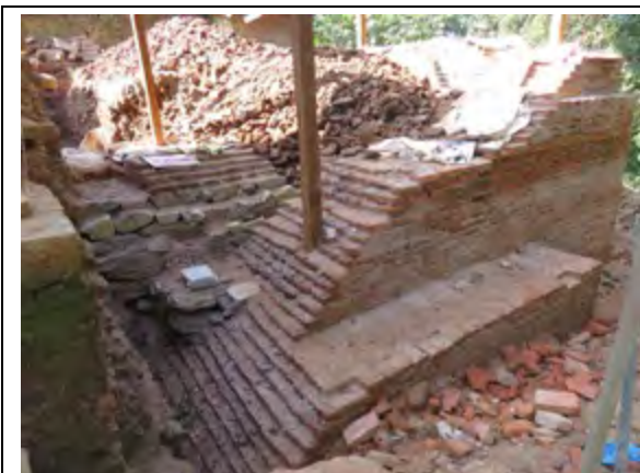
Footings of western sattal being rebuilt to stabilise top of hill
