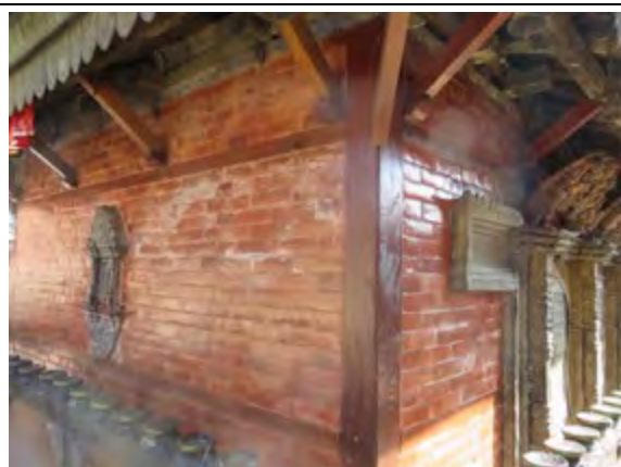
Glazed tiles have been removed from walls of Chhina Masta Temple and brickwork has been painted with a waterproof compound
