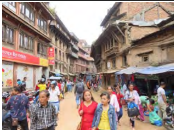
View along main path looking south - concrete framed buildings on left and traditional buildings with additional floors added on right
