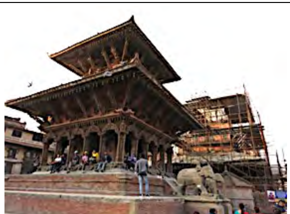
Bishwanath Temple was repaired in situ. The Bhimsen Temple is currently being repaired and rebuilt
