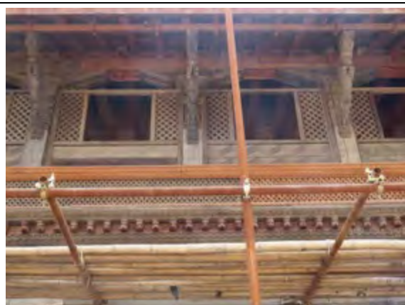
Original carved timber brackets have been reinstated.
