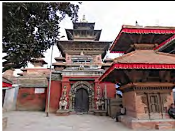
Recovery of Taleju Bhawani Temple and Mahadev (Shiva) Temple at entrance both complete
