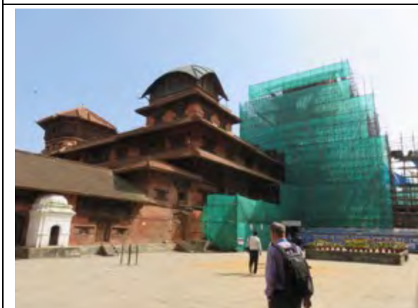
Recovery of Basantapur Durbar Palace (around Lohan Chowk) is in progress. Kirtipur Bhawan (centre) and Bhaktapur Bhawan (left) are complete. Recovery of Basantapur Bhawan (scaffolded, right) and Lalitpur Bhawan (hidden behind) are currently in progress.
