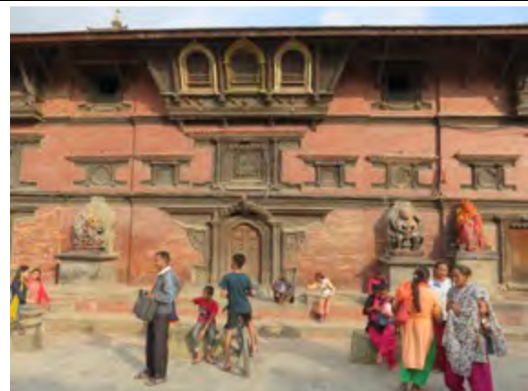
Exterior of Sundari Cok – west elevation
