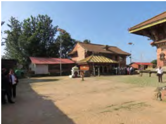
One sattal has been reconstructed on the southern side of the courtyard
