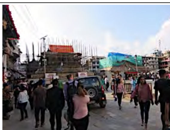
View of central section of Hanuman Dhoka Durbar Square looking west, showing reconstruction commencing on Trailokya Mohan Narayan Temple (left) and Maju Dega Temple (right), two of the tallest temples in the Durbar Square due to their being mounted on high stepped pyramidal bases.
