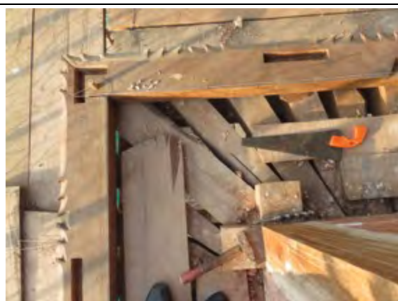
Reconstructing outer ledge of Basantapur Bhawan using traditional techniques
