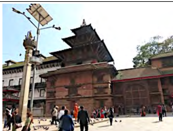
Northern face of Degutale (Degu Taleju) Temple and Shweta Bhairav Temple repaired (facing Hanuman Dhoka Durbar Square)
