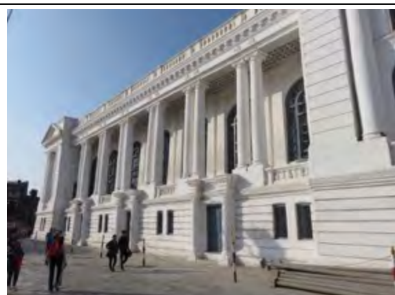
South elevation of Gaddi Baithak facing Basantapur Square
