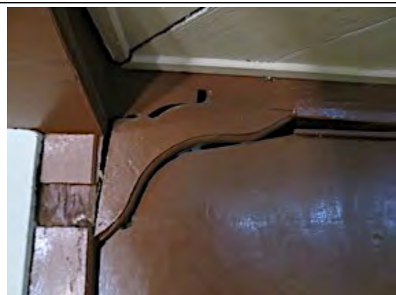
Ceiling brackets in western wing of palace
