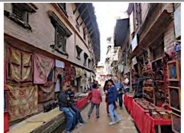
Peacock window in wall of museum reinstated (left), but wall still bulging and needing further work.
