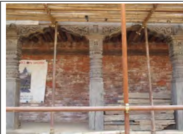
Original timber posts and carved timber brackets have been reinstated
