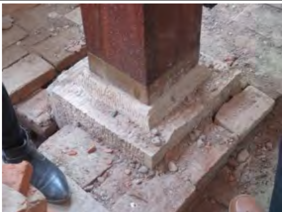
Some stone footings have been retained and others have been replaced. Copper shoes have been used to damp proof the base of the posts.
