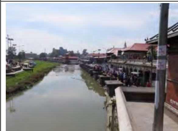
Temples, sattals and other structures along the Bagmati River have been rebuilt
