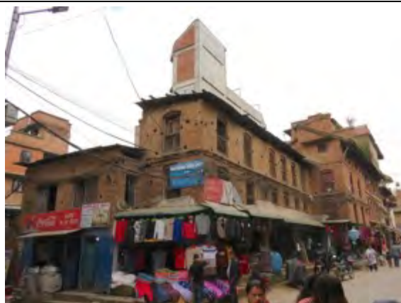
Concrete framed houses with roof terraces, stair shafts (centre) and other additions, including cantilever out over traditional roof eaves (right)
