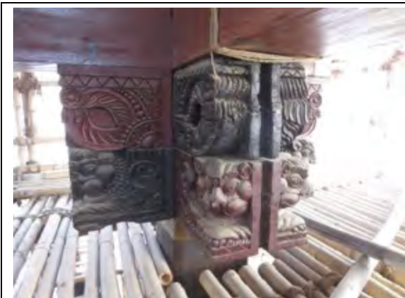
Original carved brackets repaired (original sections dark and new sections light in colour) and reinstated within second floor of new structure.
