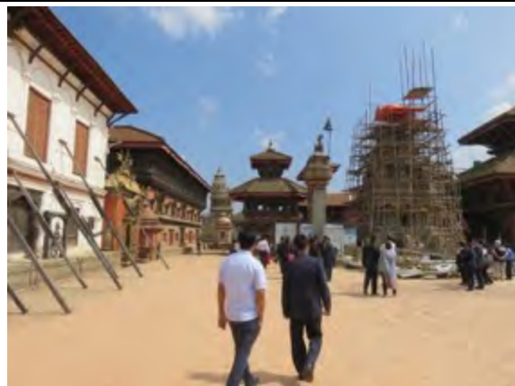
Temples at the eastern end of the Bhaktapur Durbar Square have been recovered or are in the process of recovery. Lal Baithak is on the left.
