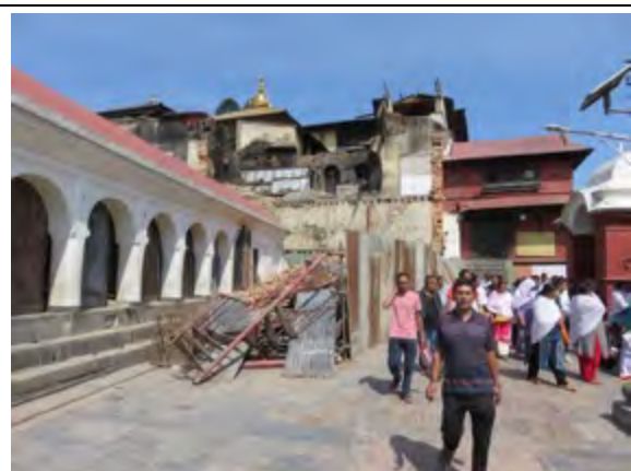
Building in main Pashupati Temple complex has collapsed since the 2017 RMM.
