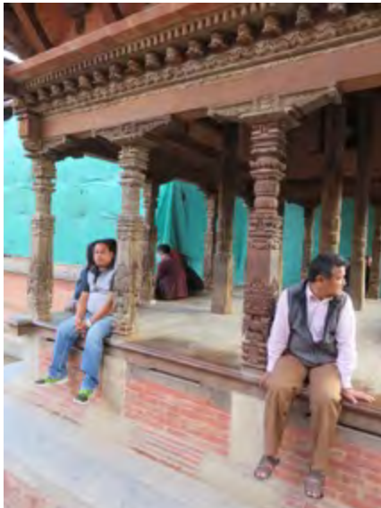
The mandapa has been rebuilt using almost all its original fabric. Only one post has been replaced.
