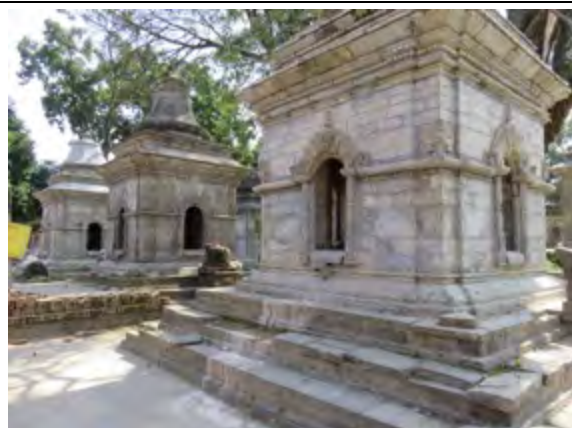
Some stone temples have been repaired
