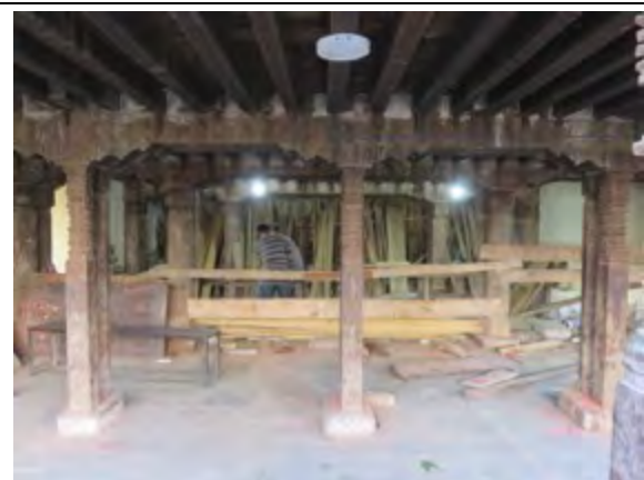
Monastery used as workshop for ongoing recovery work
