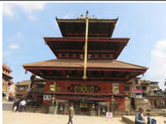
Kasi Biswanath (Bhairab Nath) Temple located on Taumadhi Square has been repaired
