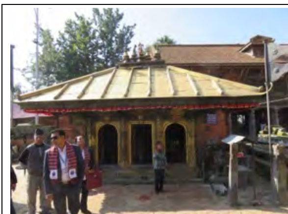
Repaired Chhina Masta Temple
