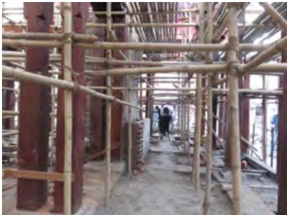
Kasthamandap during reconstruction
