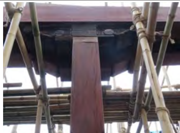
Original column bracket reinstated at ground floor level of new structure
