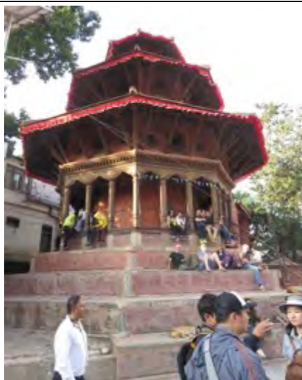
Chyasin Dega (Bamsa Gopal) has been rebuilt
