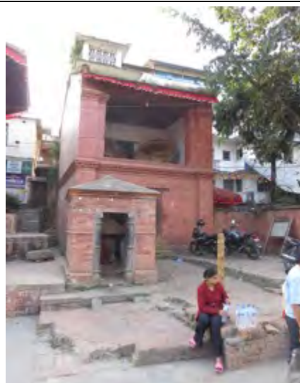
Nagara Ghar (Great Drum House) has been repaired
