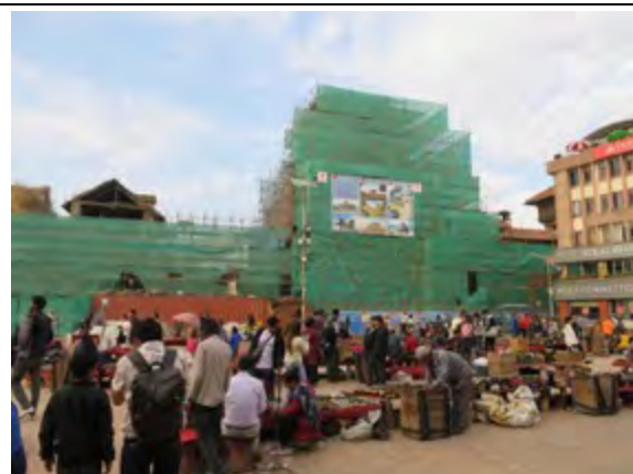
View from Basantapur Square of Basantapur Bhawan (Nine Storey Palace), currently being repaired and rebuilt
