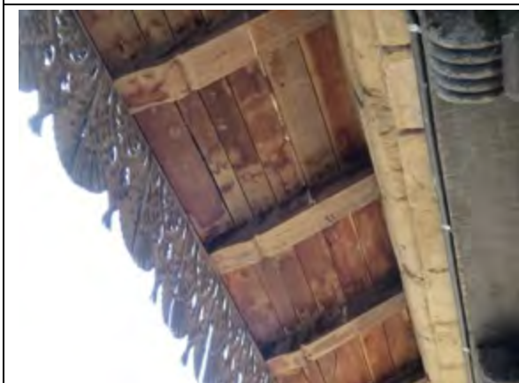
Metalwork to eaves of Santipur Temple has been reinstated
