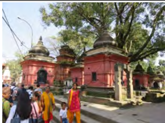
These brick temples in Gorakhnath Area have not been repaired
