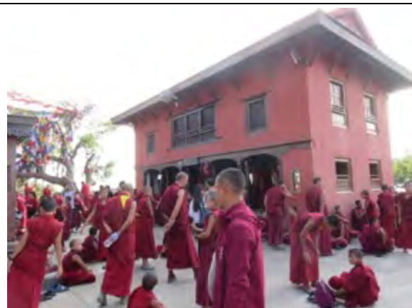
Sattal in Manjusthree (Saraswati) Area has been repaired. Annual debating festival for young monks demonstrated continuance of intangible heritage at the site.
