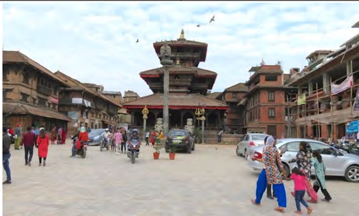
Dattatreya Square, looking east, showing traditional buildings on left and new development on right of temple. The flat roofed concrete framed building is intrusive to the square, which is part of the Protected Monument Zone.
