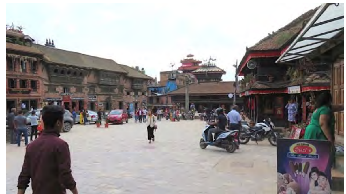
Dattatreya Square, looking west, showing traditional buildings on left and new development adjacent to and behind the temple (centre). The flat roofed concrete framed buildings are intrusive to the square, which is part of the Protected Monument Zone and KVWHP.
