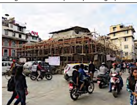
Maru Sattal (Kasthamandap) is currently being reconstructed.
