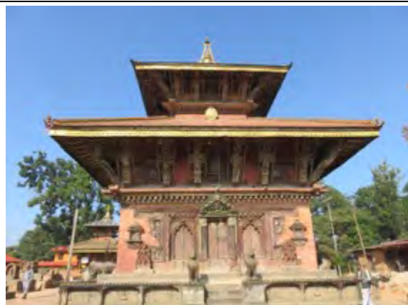
The Changunarayan Temple has been repaired and strengthened.
