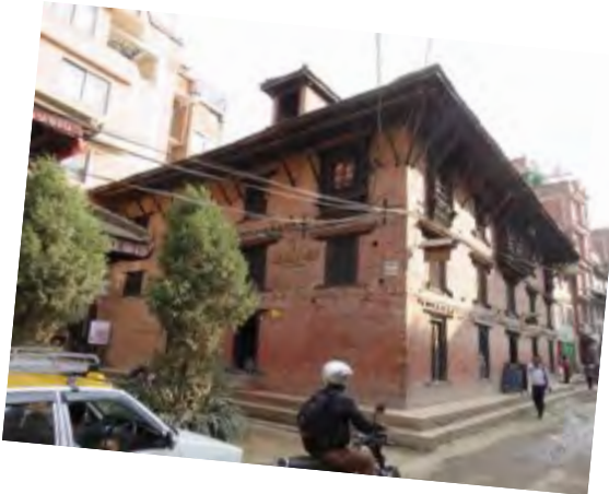
Traditional refurbished as a guesthouse in the Patan buffer zone
