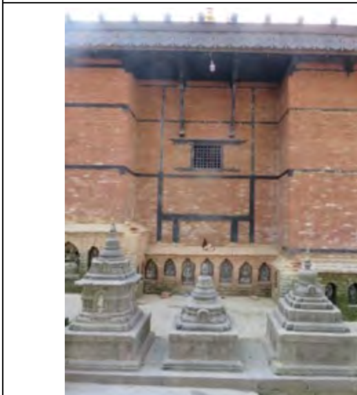
Timber bands have been incorporated into the masonry walls
