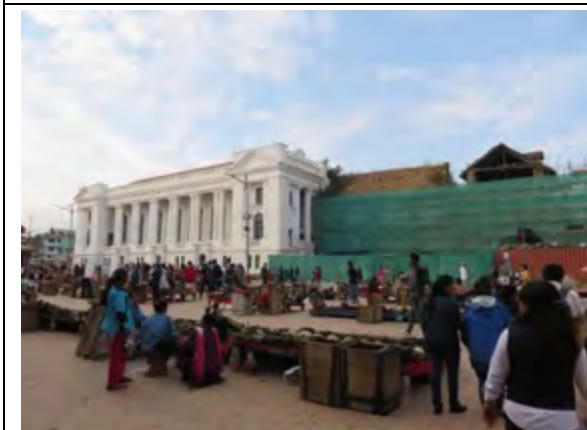
View from Basantapur Square of Gaddi Baithak and southern wing of palace (partially demolished behind scaffold)
