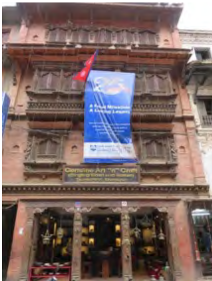
Modern concrete framed building with brick façade and detailing to replicated traditional house in accordance with building bylaws
