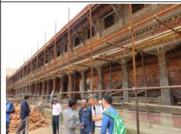
Reconstruction of the sattal incorporating as much original timber fabric as possible.
