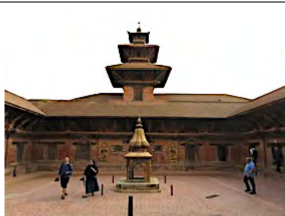
Temple over Sundari Cok damaged in earthquake has been repaired
