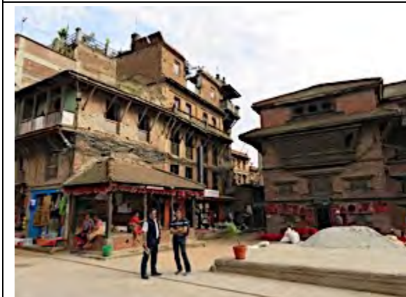
Traditional houses at eastern end of Dattatreya Square severely damaged or collapsed – being replaced with concrete framed buildings.
