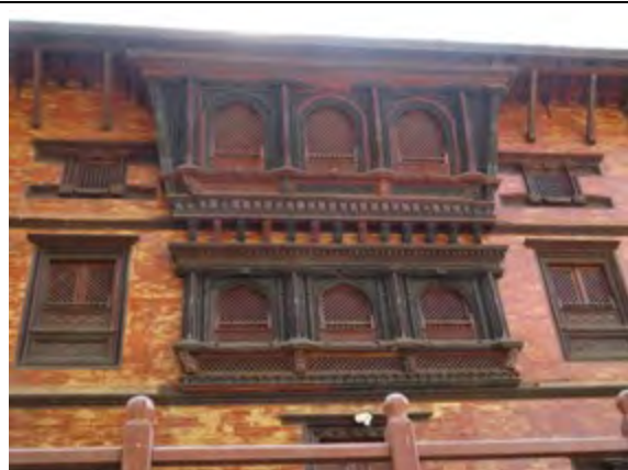
Detail of reconstructed building in Guheshwori Temple complex showing water proof compound applied to surface of bricks. Windows have been repaired – original timber is dark and new timber is light in colour.
