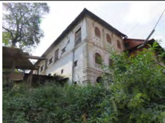
Rana style building at eastern end of Guheshwori Temple complex has not been repaired as yet
