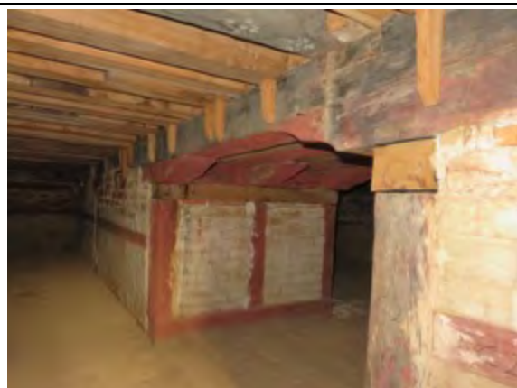
Inside Basantapur Bhawan showing traditional pegging of floor
