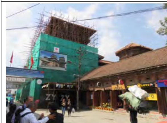
Lalitpur Bhawan scaffolded and recovery in progress.
