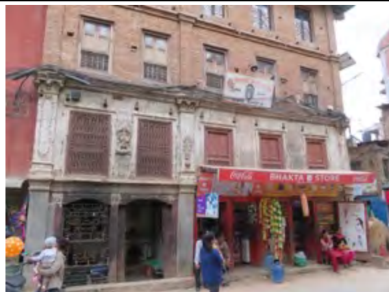
Early twentieth century rendered façade on main path, which should be considered for protection
