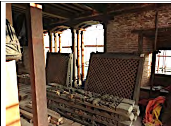
Inside Basantapur Bhawan (Nine Storey Palace) – carved brackets and timber screens repaired and ready for reinstatement
