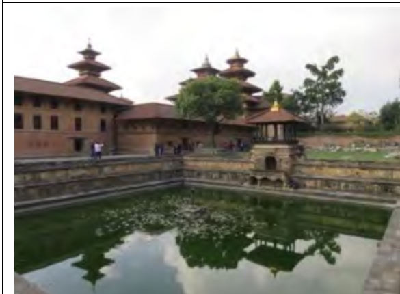
View over Bhandarkhal Tank, looking north. The rear wall of Sundari Cok (left) collapsed during the earthquake and has been rebuilt
