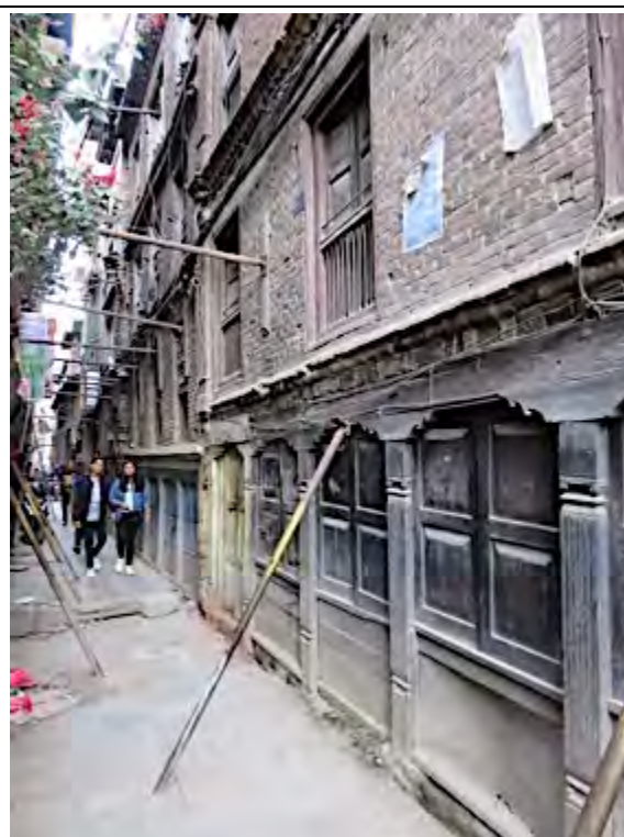
Housing and other historic structures are braced off each other to prevent them from falling – along southern boundary of the Hanuman Dhoka Durbar Square Monument Zone
