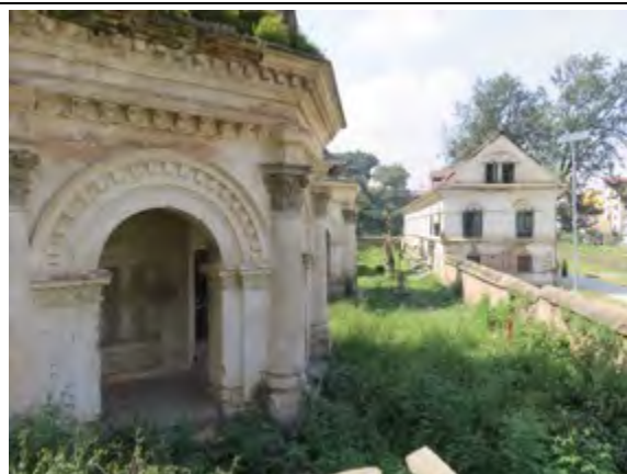
Detail of reconstructed building in Guheshwori Temple complex showing water proof compound applied to surface of bricks. Windows have been repaired – original timber is dark and new timber is light in colour.
