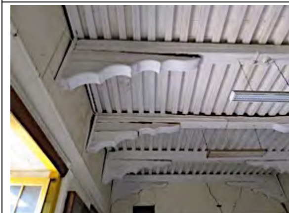
Timber ceiling brackets in Lal Baithak
