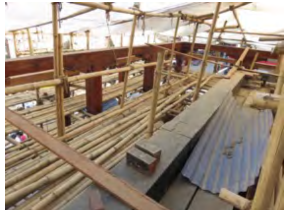
Kasthamandap – original beams reinstated (dark)
