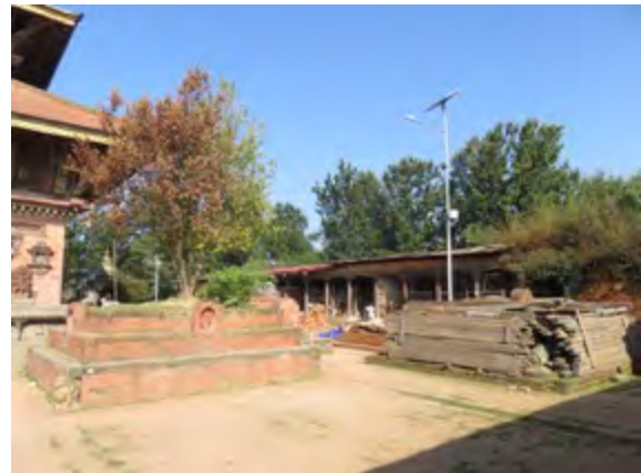
The sattal on the northern side remains in a dilapidated state.
