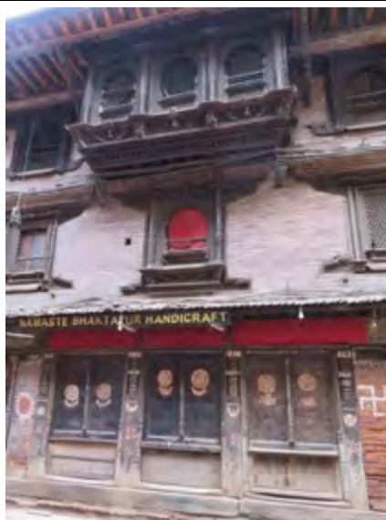
Traditional house has been repaired
