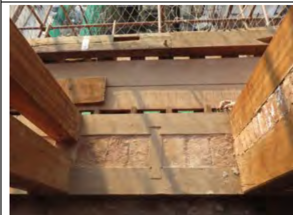
Traditional jointing detail sed in repairs to timber and brick structure of Basantapur Bhawan. New and old timber pieces pegged together in outer beam.
