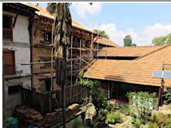
Rear wing of museum which is currently being rebuilt
