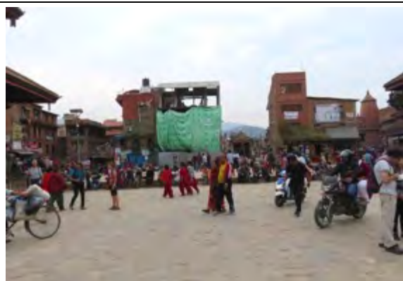
Buildings lost on the southern side of Taumadhi Square are being replaced by concrete framed buildings.
