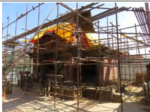
Jayabageshori Temple is currently being repaired
