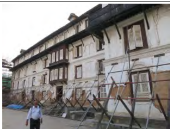
Central portion of palace is yet to be repaired (facing Nasal Chowk)
