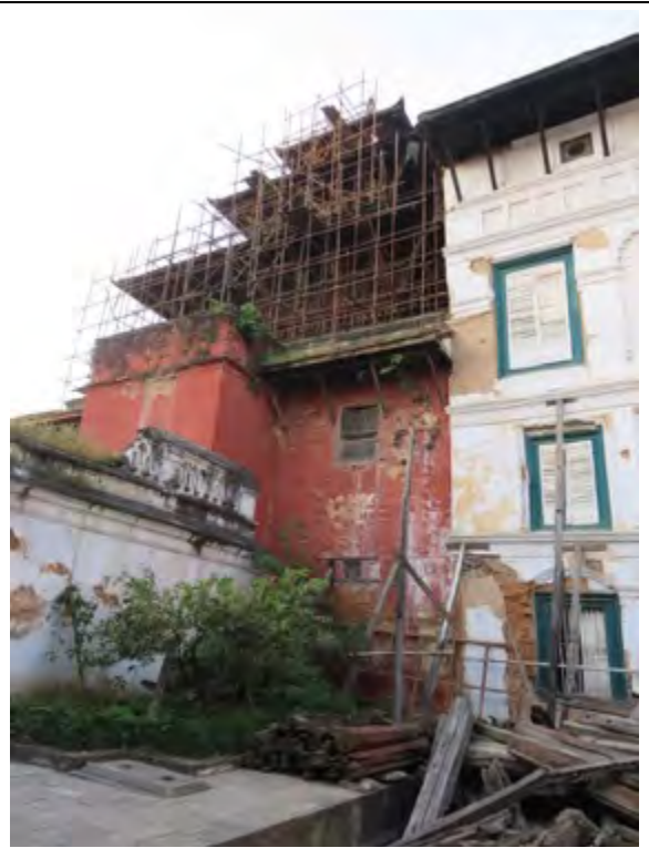
Southern side of Degutale Temple still scaffolded facing palace Dakih and Masan Chowks
