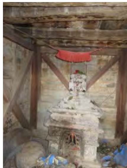
A braced timber frame has been built around the central shrine to provide some protection to the shrine and to provide some seismic strengthening to the structure
