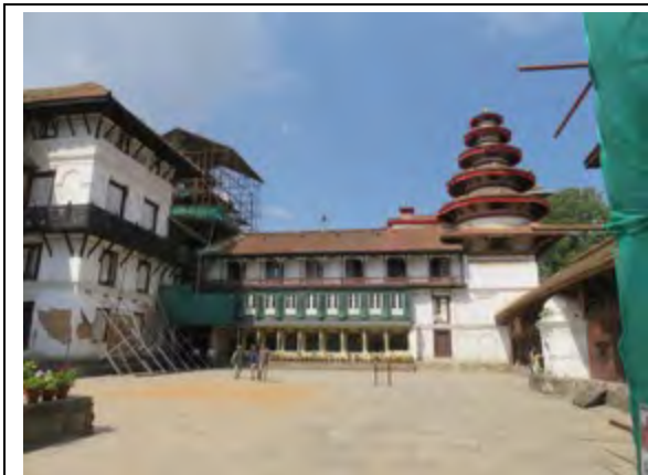
Northern portion of Hanuman Dhoka Durbar Palace viewed from Nasal Chowk has been repaired, including Panchamukhi Hanuman Temple (right).
