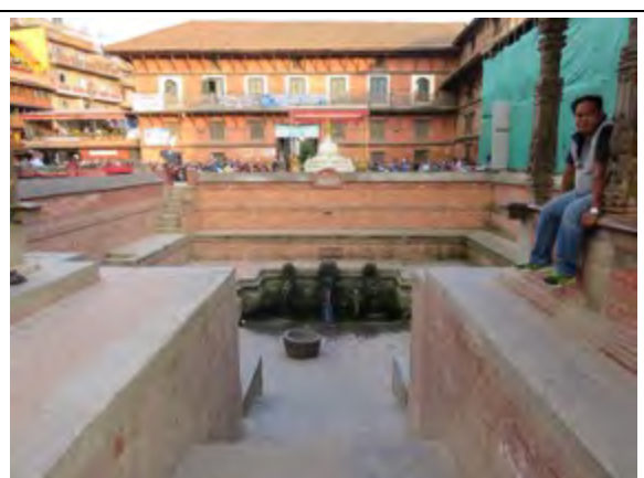
Manga Hitti with Bahadur Shah wing (north wing) of palace (now a school) behind. This wing has been repaired. The section of the palace on the right is currently being repaired.
