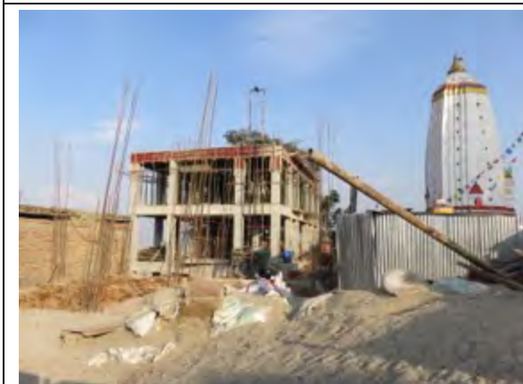
New monastery to replace buildings destroyed in earthquake is under construction
