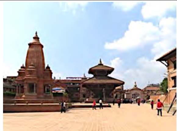
Temples in western end of Bhaktapur Durbar Square repaired and/or reconstructed.
