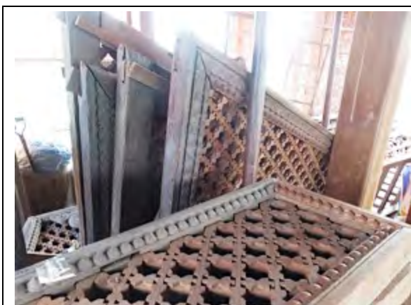
Repaired timber screens for reinstatement on Basantapur Bhawan
