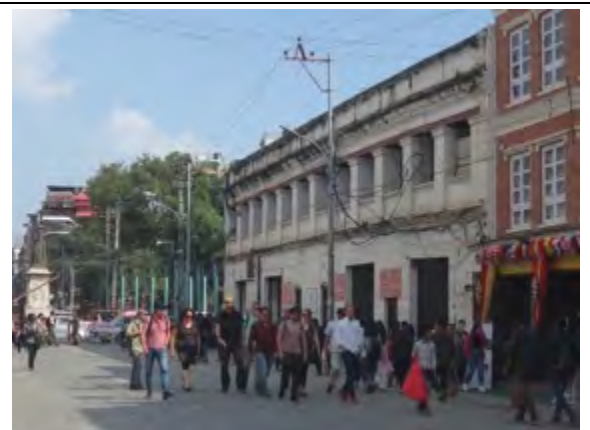
North elevation of the fire station facing the Ganga Path. This building is located within the protected monument zone.
