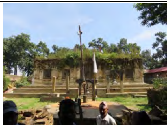
Remains of the domed Vishwarupa Temple on top of the hill. Further collapse and dismantling has occurred since the 2017 RMM.
