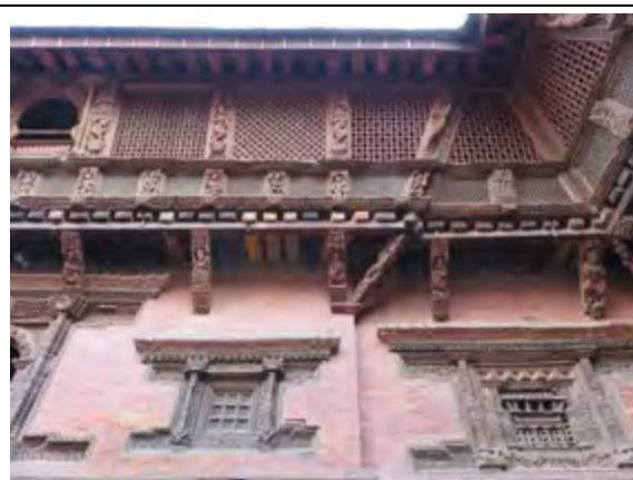
Detail of timber repairs
