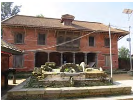
Rebuilt Amatya Sattal
