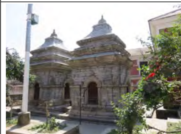
Temples near Bagmati River have been rebuilt using original and new stone
