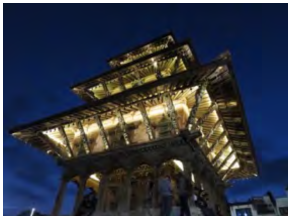
LED lighting being tested on Hari Shankar Temple, which has been repaired and rebuilt.
