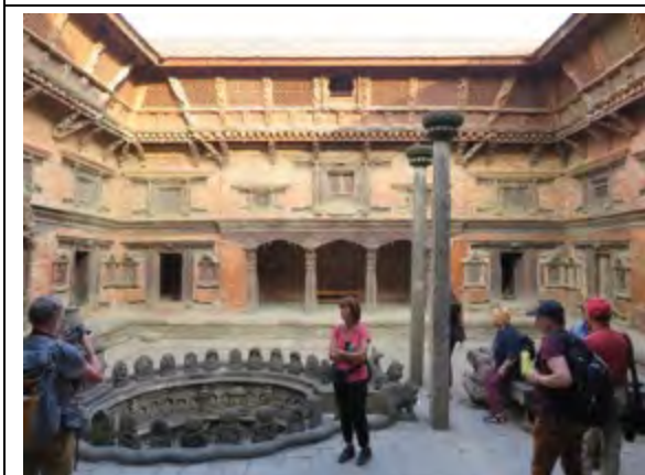
Eastern wing of Sundari Cok has been rebuilt, reinstating original fabric salvaged following the earthquakes
