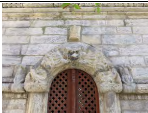
Lime mortar with stone dust has been used in the reconstruction
