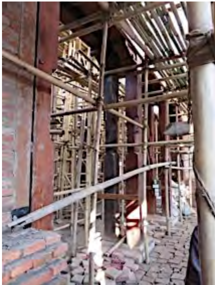
Kasthamandap – Original post (dark) reinstated amongst new posts (light). Old bricks have been salvaged and reused in brick plinth.
