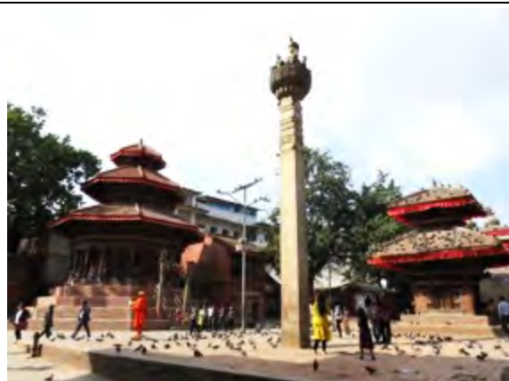
Pratap column (centre) has been repaired and re-erected. Chyasin Dega (left) and Laxmi Narayan Temple have been repaired – northern section of Hanuman Dhoka Durbar Square, looking north.
