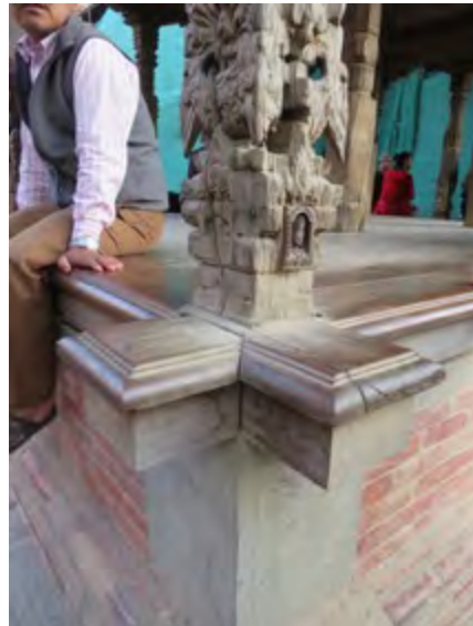
Detail of mandapa post and floor connection.
