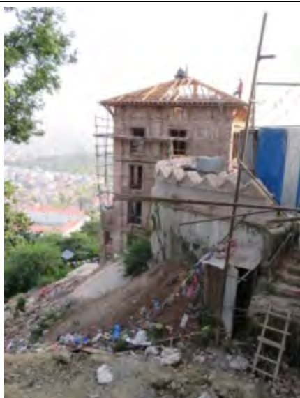
Building at top of eastern stairs is being rebuilt
