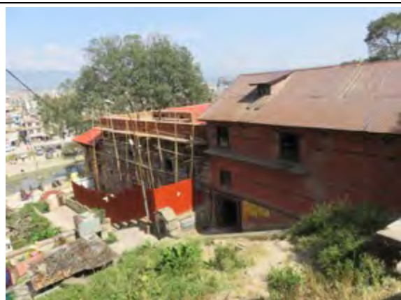
Guheshwori Temple complex in process of being rebuilt. This is occurring in stages.
