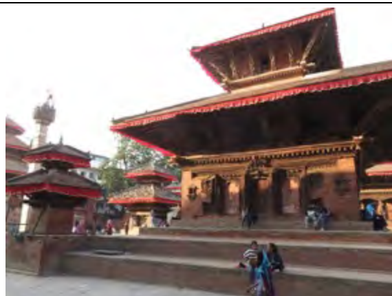
Jagannath Temple has loose bricks in upper storey, but people are still occupying area beneath as safety barriers have been removed
