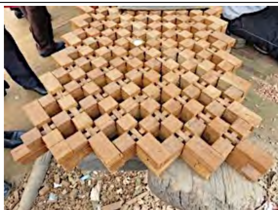
Lattice screens are being remade using traditional techniques
