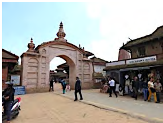
Khauma Gate (western entrance gate) to Bhaktapur Durbar Square reconstructed.
