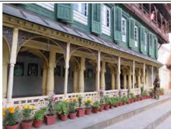
Southern façade of northern portion of Hanuman Dhoka Durbar Palace repaired and conserved
