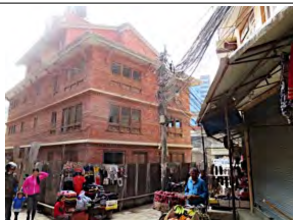
New brick clad concrete framed building in buffer zone
