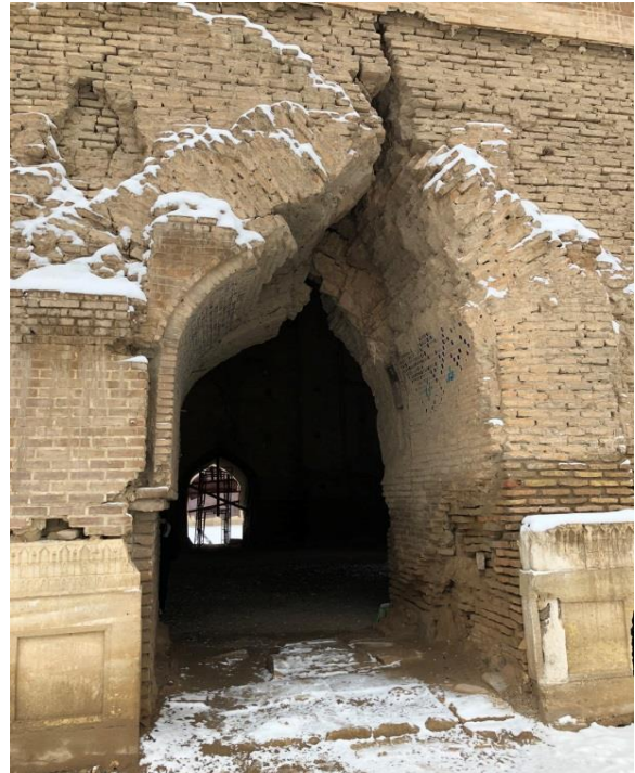
Bibi Khanoum: evidence of structural failure and the need for major conservation works.
