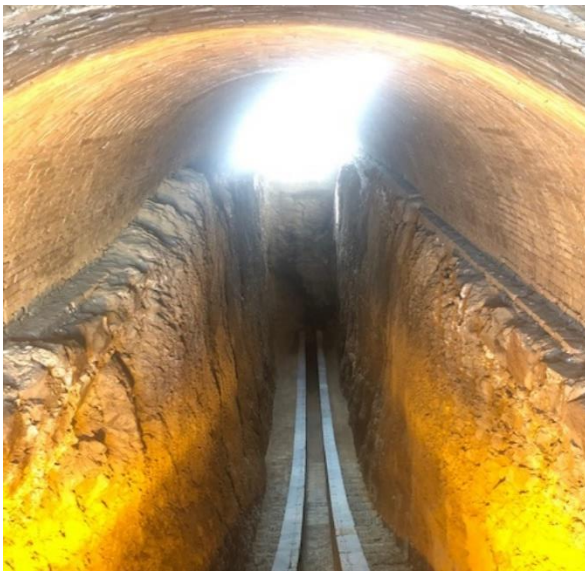
Underground giant astronomical 'sextant' device at Ulugh-bek's Observatory.
