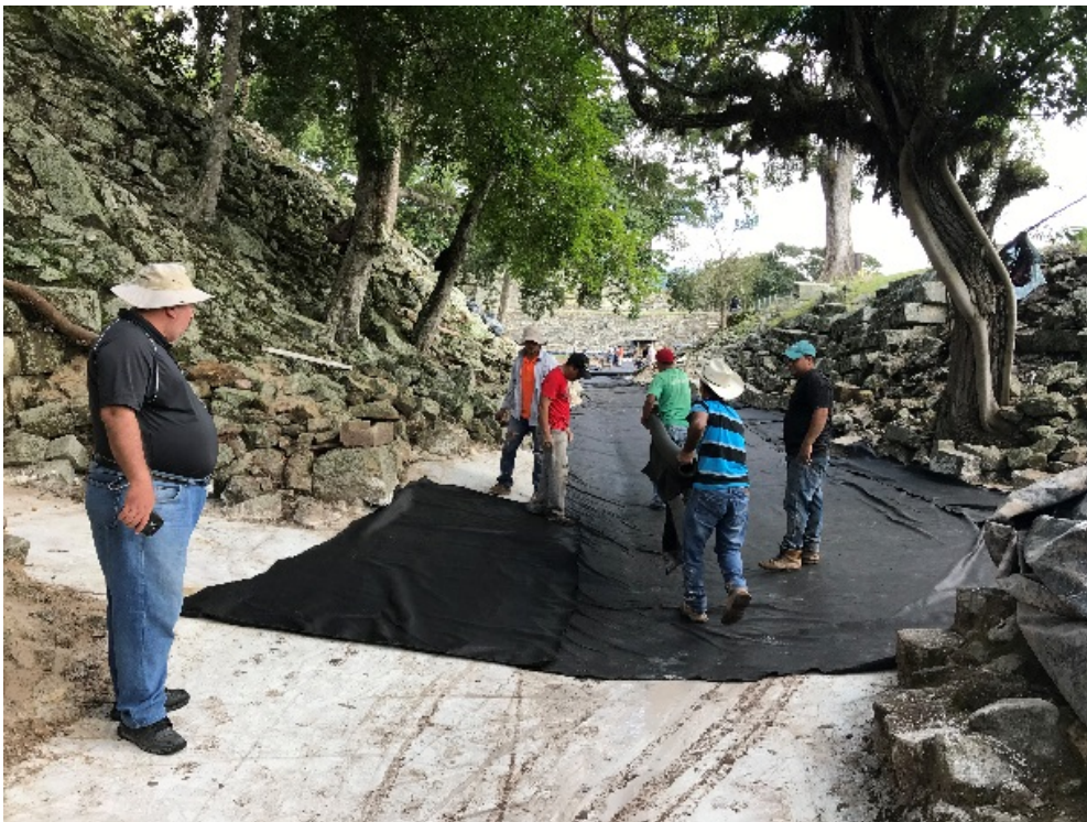
Figure3: The waterproof geo-membrane above a layer of sand, gravel and lime.
