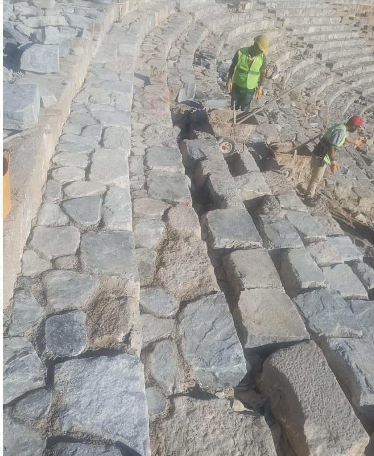
Rubble stone implementations in the sections consisting of large rough cut stones
