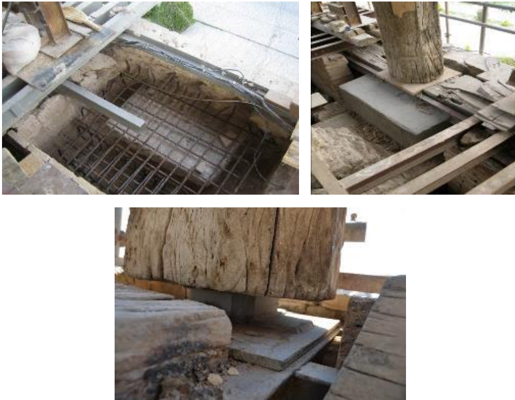
Figure 20. Ali Qapu edifice, strengthening the supports of the columns (2005 to 2017)
