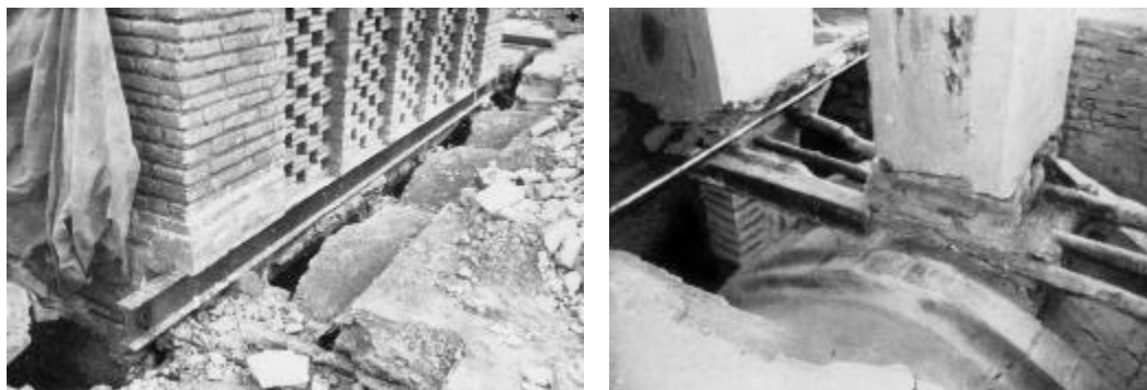
Figure 12. Ali Qapu edifice, lightening the roofs at sixth floor, 1965-1970
