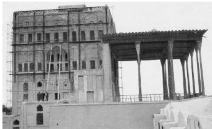
Figure 14. Ali Qapu edifice, using horizontal circumferential frame in the whole building in order to prevent the external parts from detaching, 1964-1970
