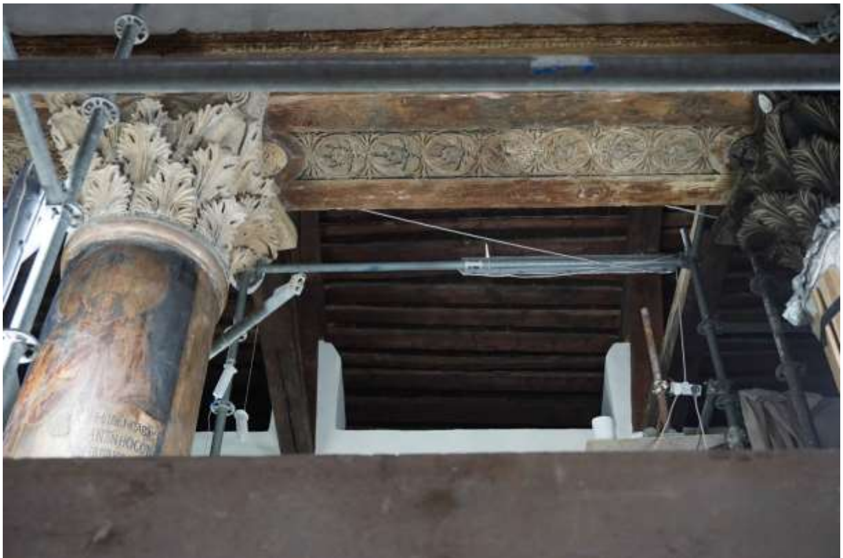
5.16 Nave capitals, architraves and soffits after cleaning
