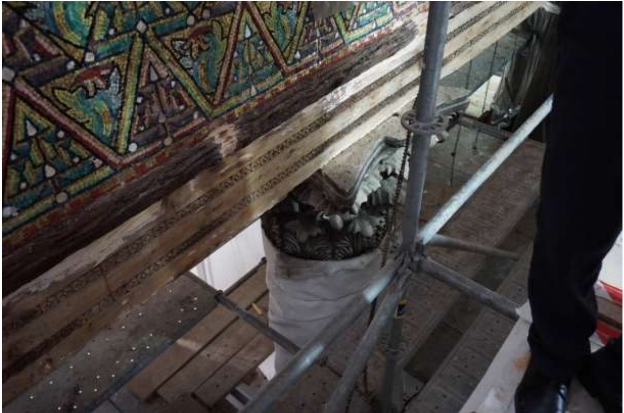
5.15 Nave architraves and mosaic during cleaning
