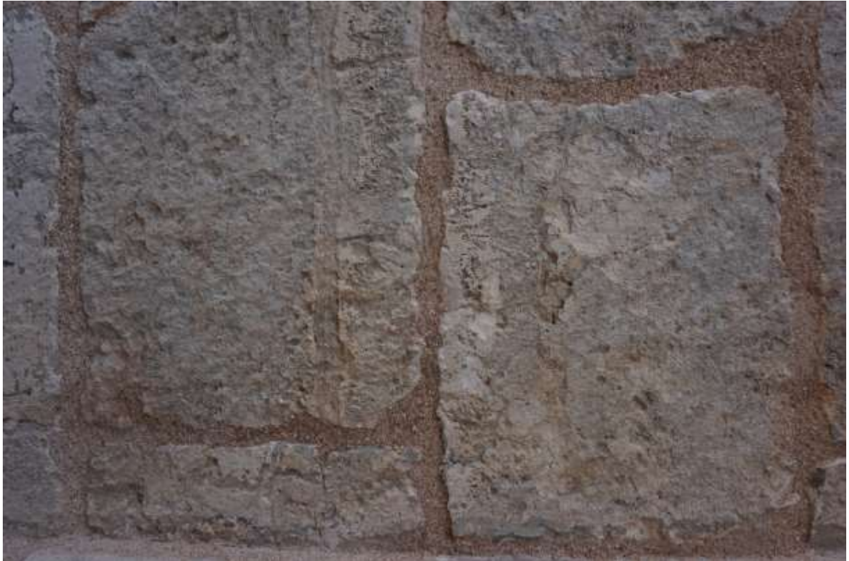
5.8 Repointed stonework to external high level elevations
