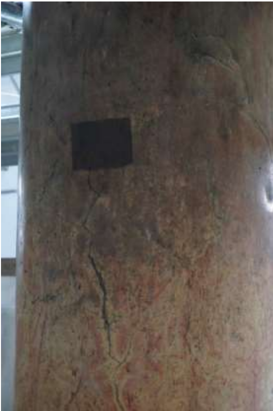
5.13 Nave columns cleaned with uncleared patch
