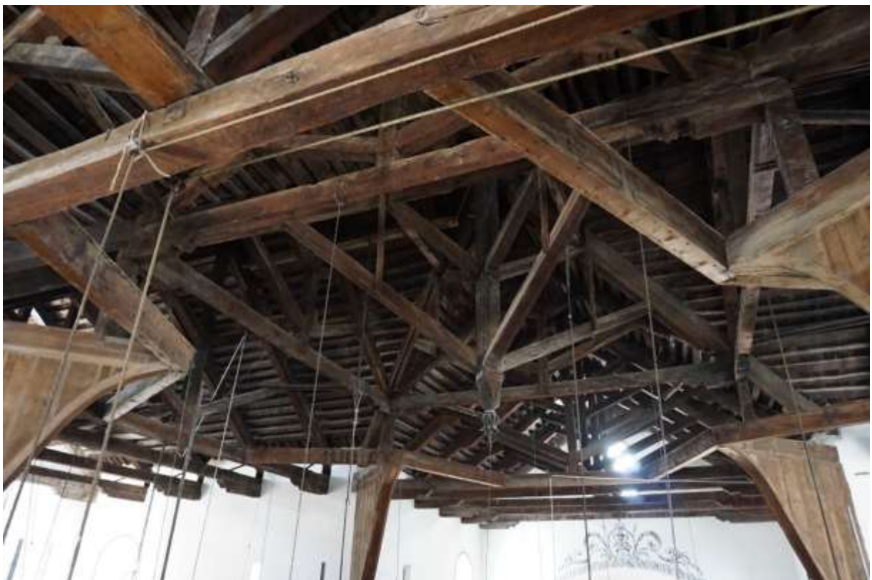
5.2 The repaired roof
