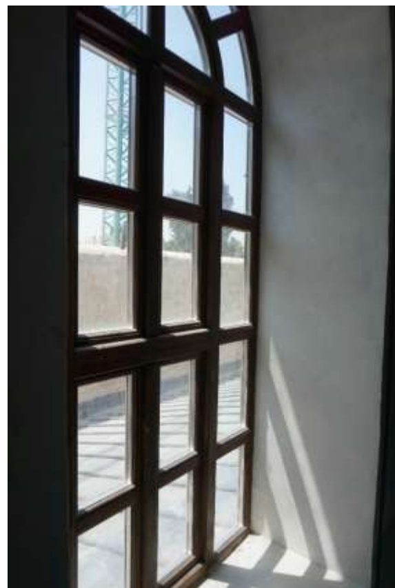
5.5 New double-glazed clerestory windows
