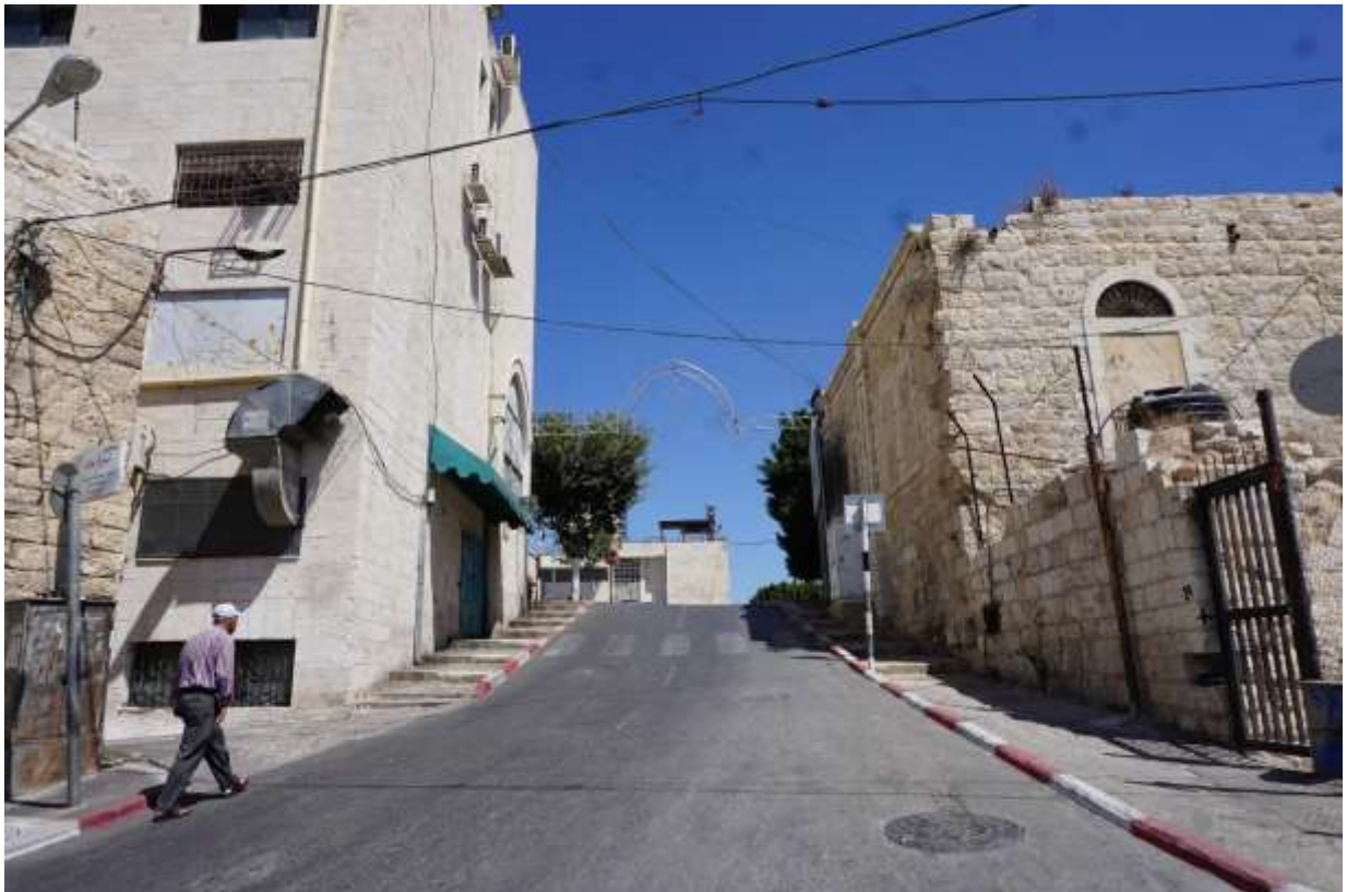
5.22 Location of proposed exit from the Manger Square Tunnel, Armenian Patriarchate car park to the right, buildings behind and to the right would be demolished
