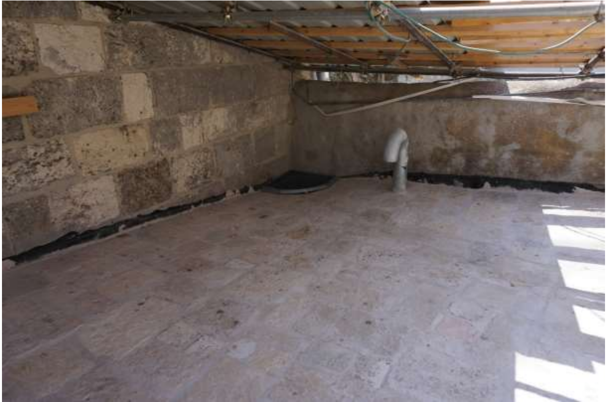
5.6 Relaid narthex roof stone paving over waterproofing layer
