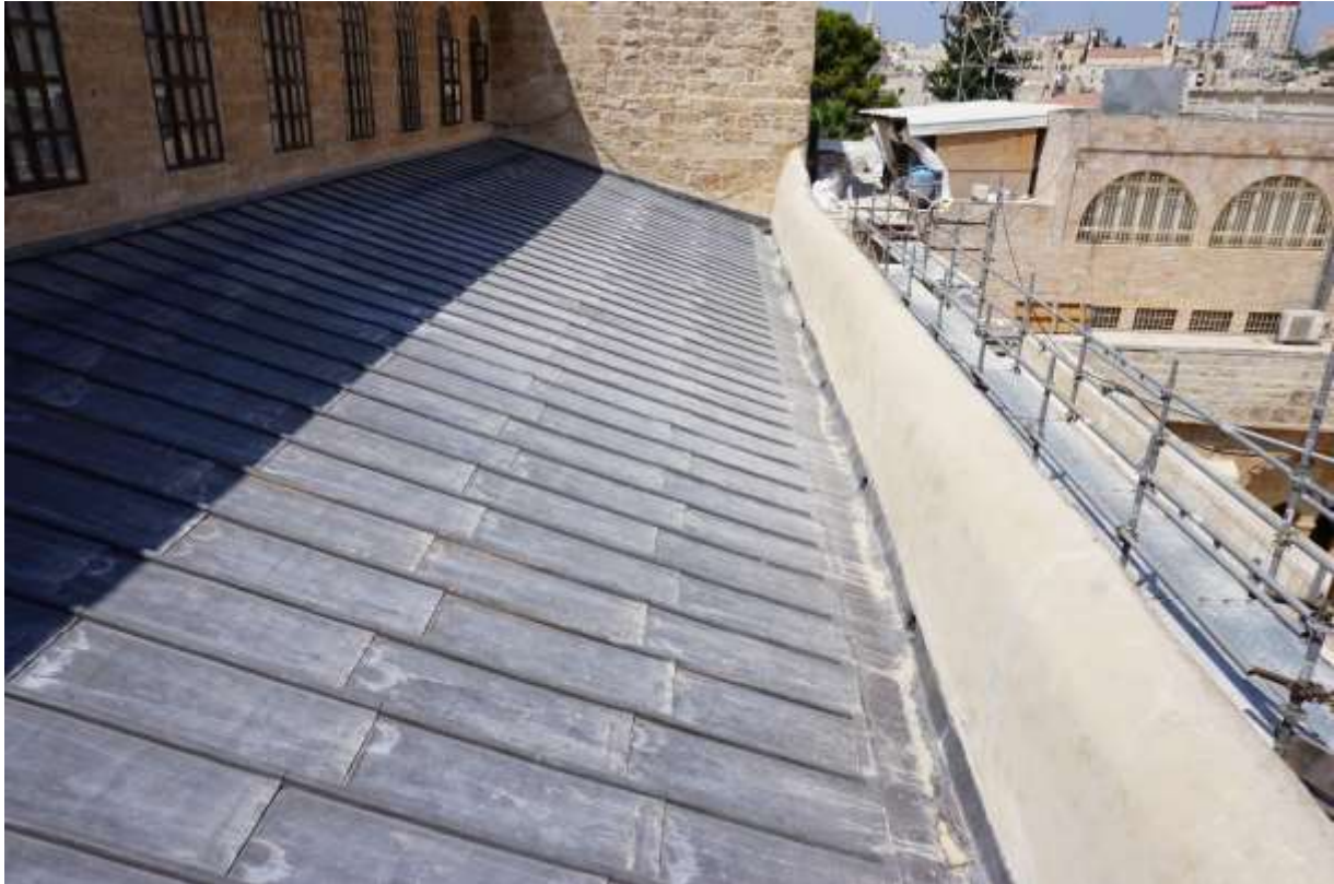
5.3 Re-leaded aisle roofs with reopened rainwater outlets
