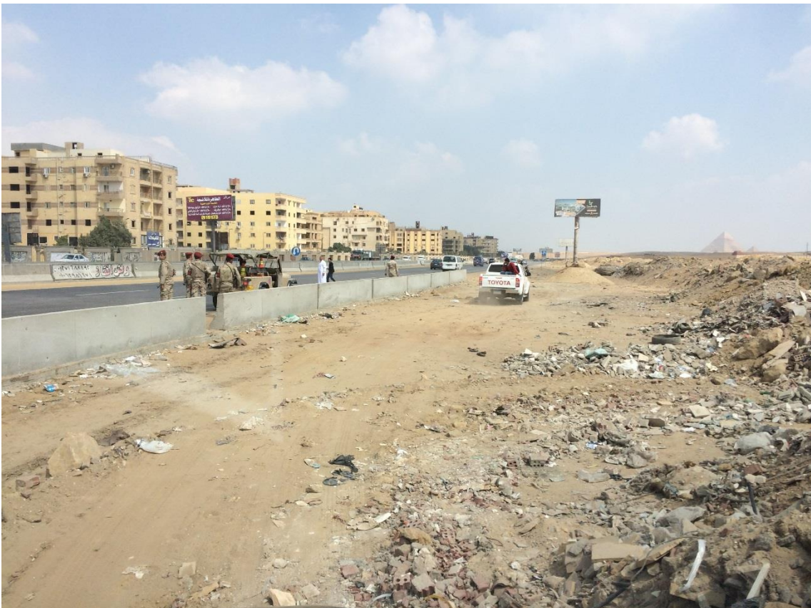
El Faiyum-Desert Road with section of concrete barriers
