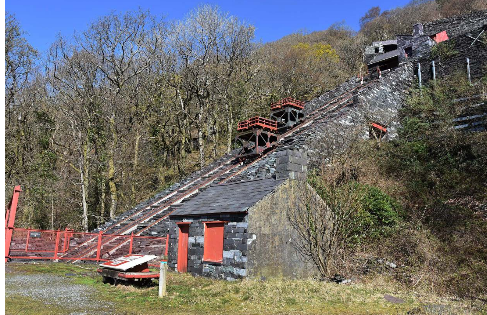
The V2 inclined plane at Vivian quarry (Component Part 2) has been conserved and returned to working order as part of the National Museum © Crown copyright: RCAHMW.
