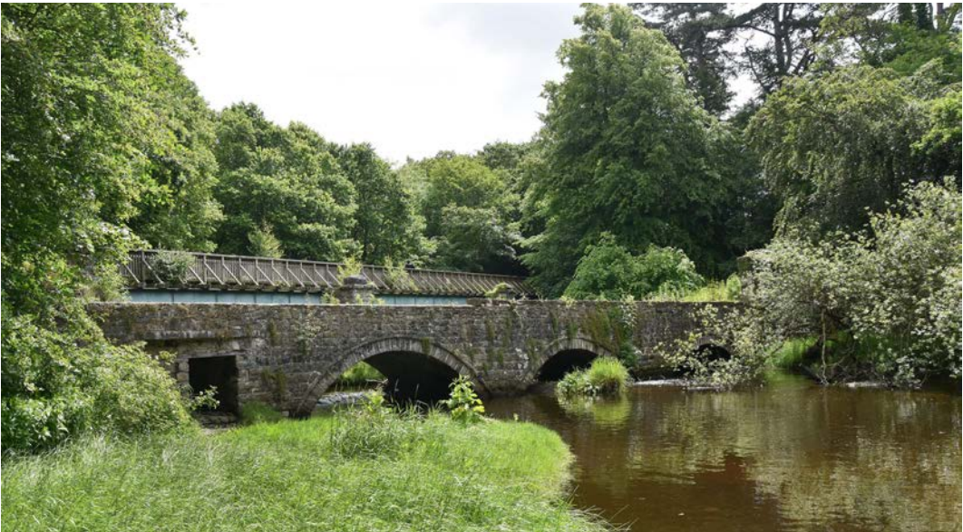
The Cegin viaduct (Component Part 1) was built to carry horse-drawn slate trains over the river and is one of the oldest surviving multi-arched railway bridges in the world © Crown copyright: RCAHMW.
