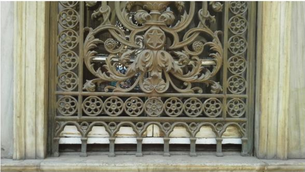
12. The sabil and annexes restored but empty
