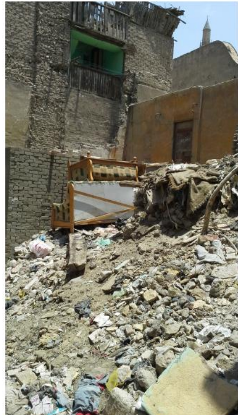
18. Demolitions in Al-Hattaba
