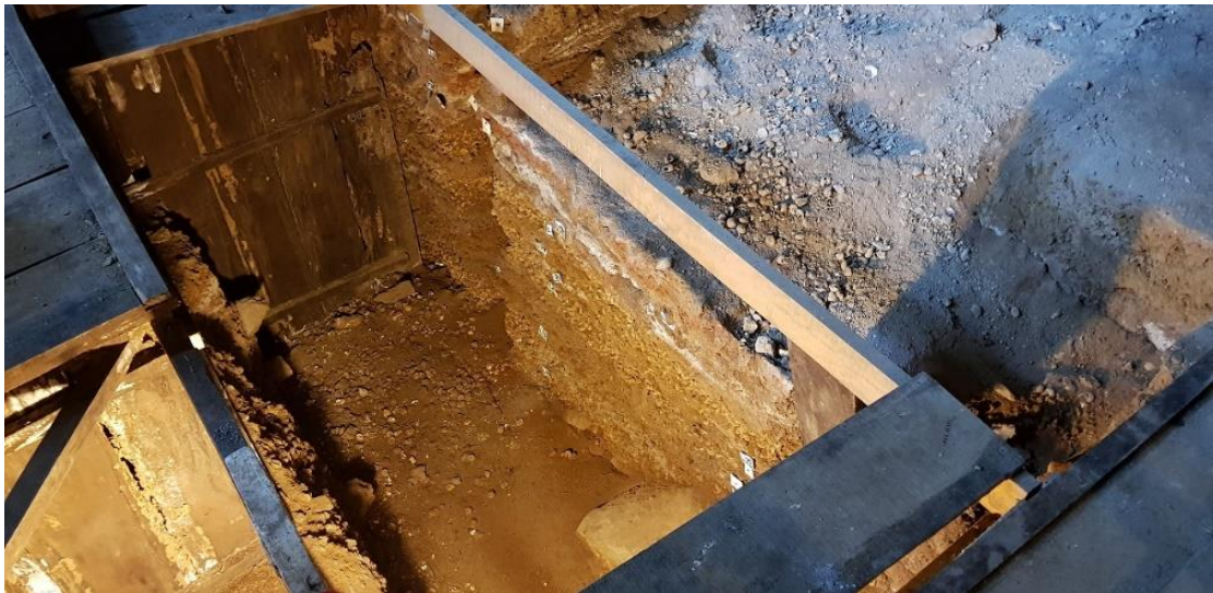
© Andrew Sneddon, 2019 – The trench has not been backfilled, although it is supported with timber beams and appears in good condition.
