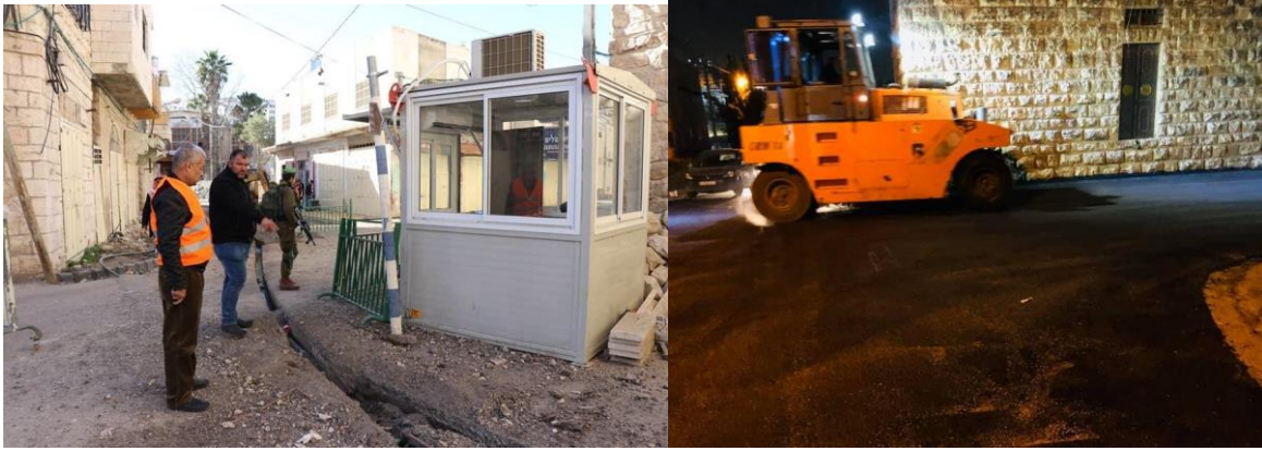
Rehabilitation of infrastructure in the buffer zone of WHP
