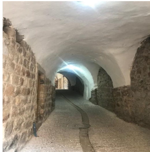
Rehabilitation of infrastructure in the
