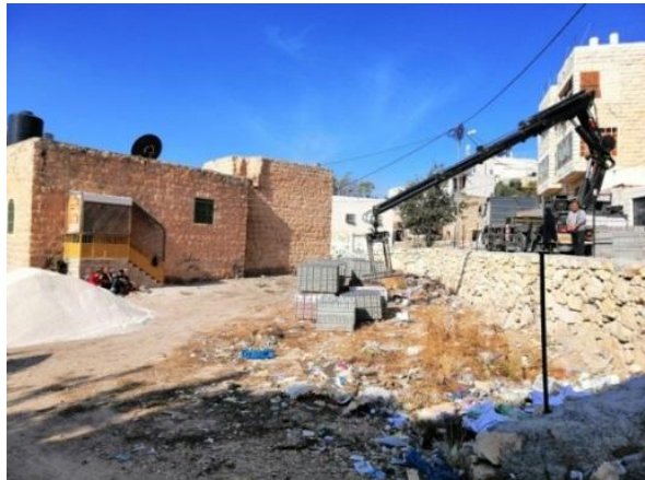
Al-Emar playground before and after rehabilitation
