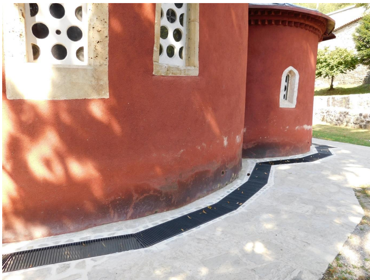
3. Drainage system around the churches of the Patriarchate of Peć, August 2019.
