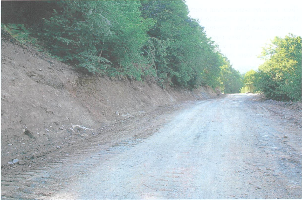
3. Main road construction near the Dečani Monastery, August 2020
