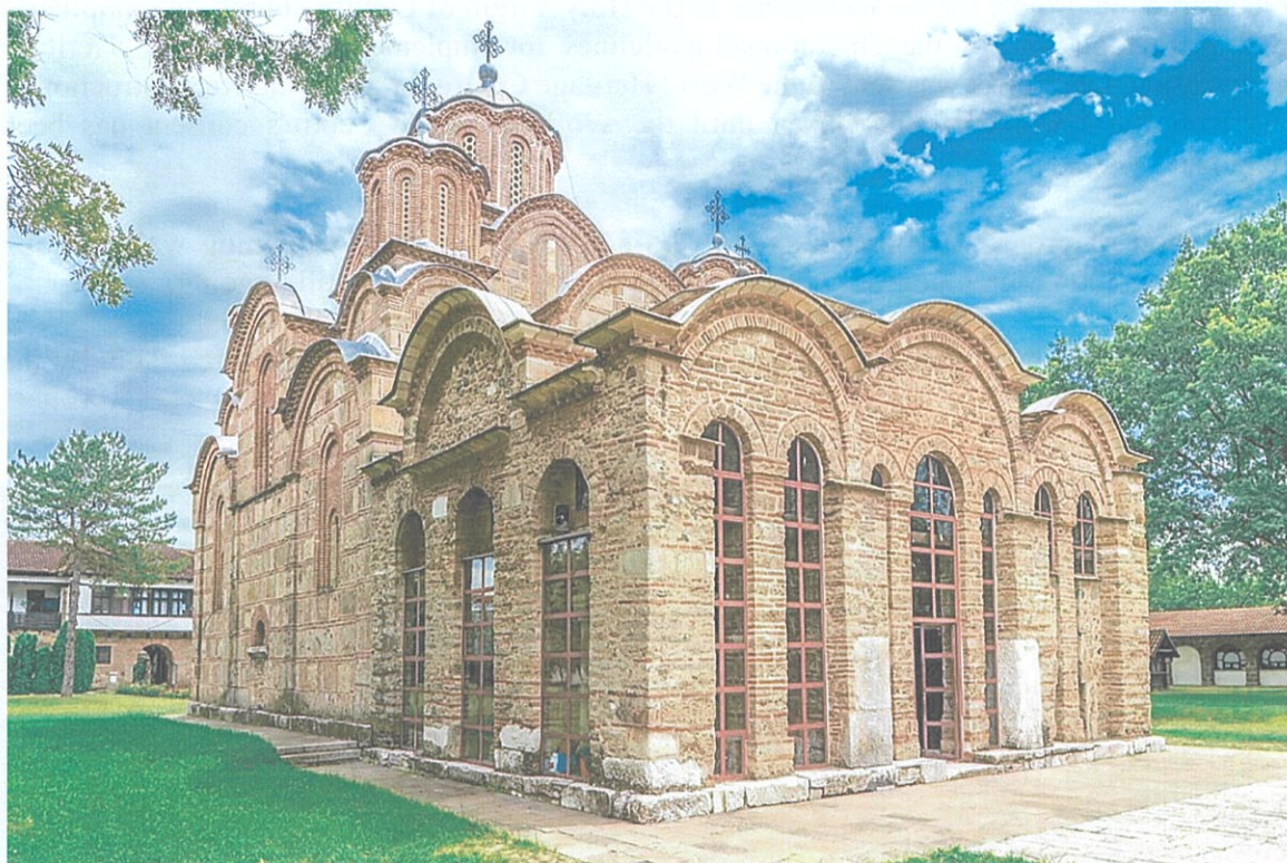
6. Southwestern view of the church in Gračanica, June 2020.
