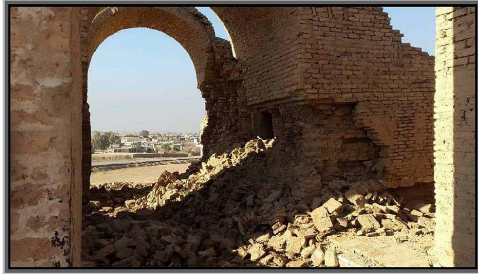
Fig. 3: An image of the vandalism of the gate by ISIS.
