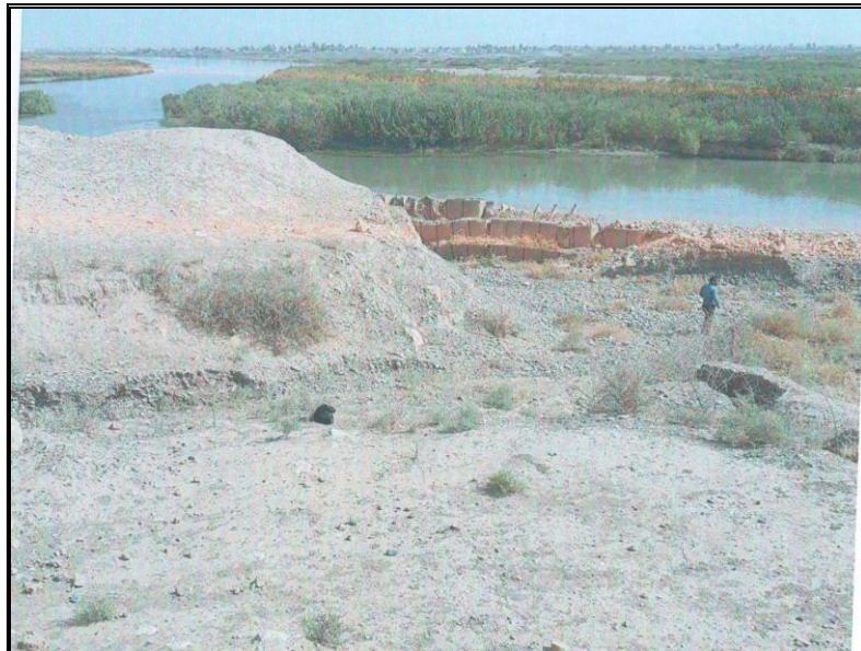
Figure 6 The valley formed by rainwater that led to the fall of the retaining wall stone.
