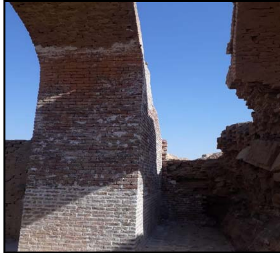
Fig. 4 conservation work performed by the team at Tabira Gate in 2020 season (Source: Department of Antiquities of Sherqat, 2020)
