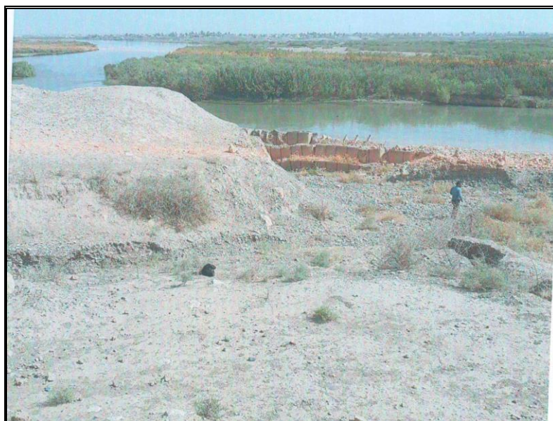
Figure 6 The valley formed by rainwater that led to the fall of the retaining wall stone.
