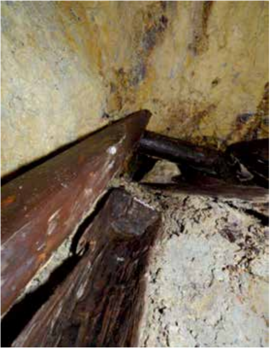
14. Launder (wooden water-channel) that received water from the still adjacent remains of the upper waterwheel in Cătălina Monulești Mine. (© Călin Tămaș)
