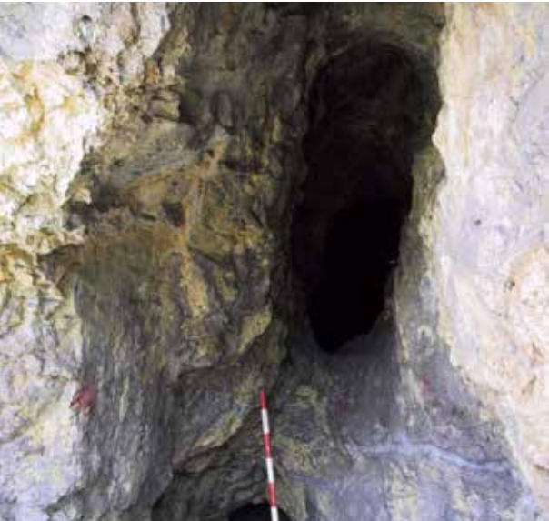
27. Cetate - Găuri Area: Roman works opened with fire and water (MNIR Archive)
