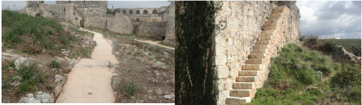
Rehabilitation works to the short visitor route.
