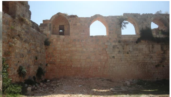
The byzantine wall on the southeastern side of the castle - after
