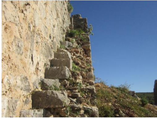
The stone step before restoration
