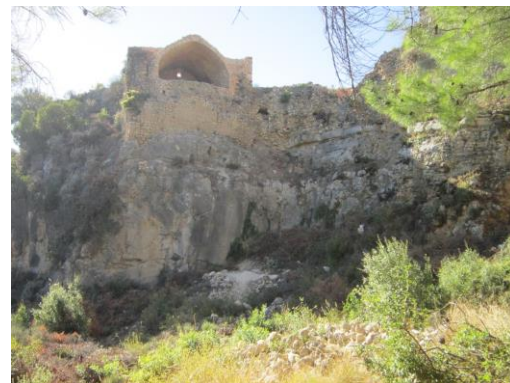
The damaged tower after restoration
