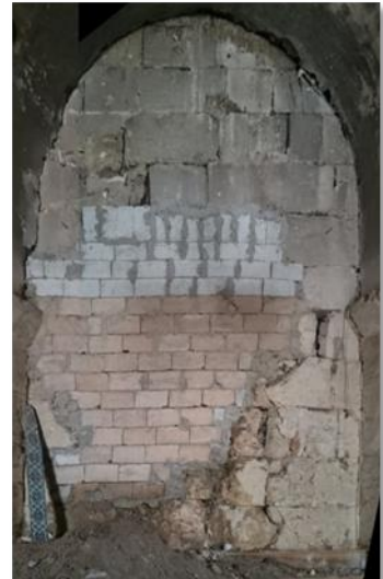
The restoration work in the Qibla in the mosque's includes documenting, dismantling, reconstructing and treating walls and columns, including cleaning and treating holes, filling mortar, and stone hammering.
