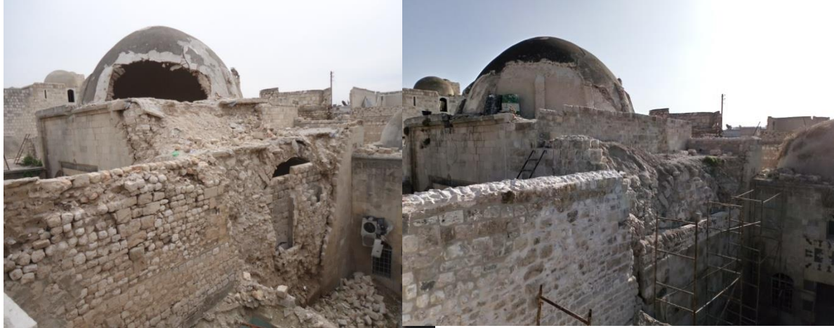
The dome of the Southern Iwan before and after the restoration
