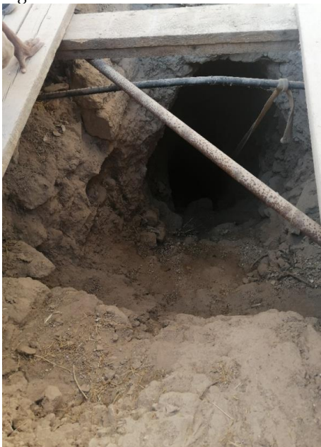
Before filling the existing tunnels
