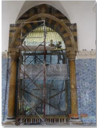
Maintenance and restoration of the shrine of the Prophet Zakaria included the manufacture of missing Qashani tiles for its internal and external facades and the maintenance of the old copper frames.
