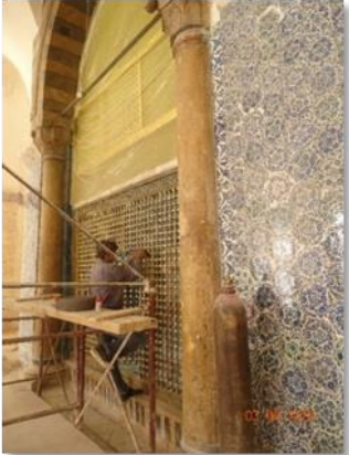
Maintenance and restoration of the shrine of the Prophet Zakaria included the manufacture of missing Qashani tiles for its internal and external facades and the maintenance of the old copper frames.
