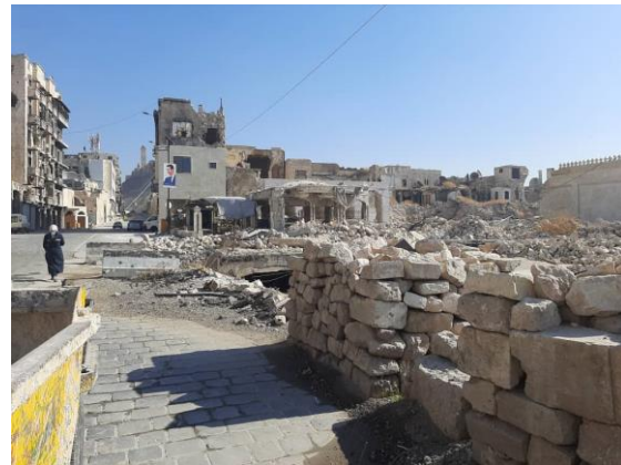
The damage at the Al-Niswan Souk
