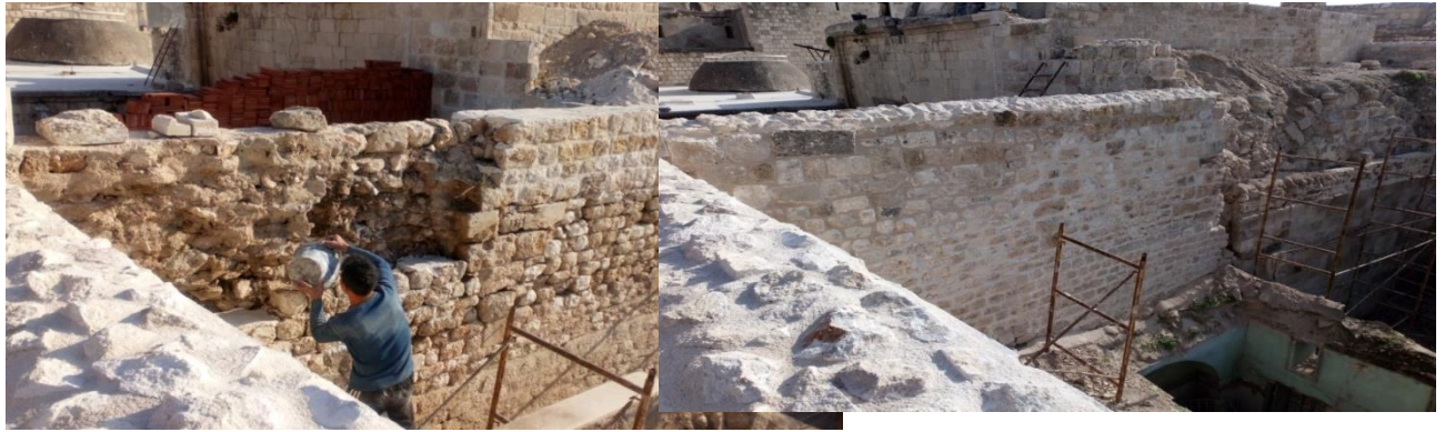
Restoration of the damaged stone walls during and after
