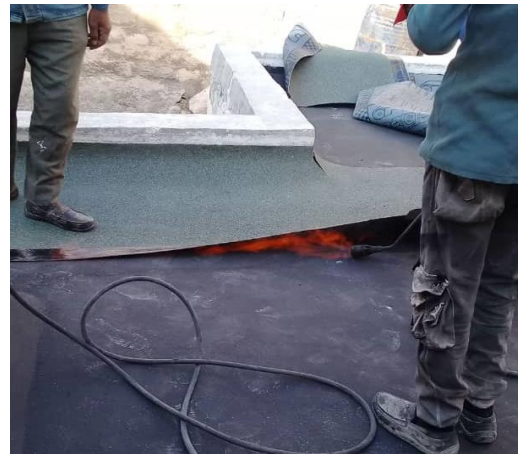
Implementing a moisture isolation layer to the roof
