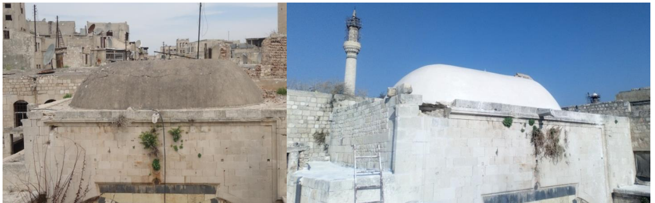
Painting by the lime mortar to the external surface of the domes before and after
