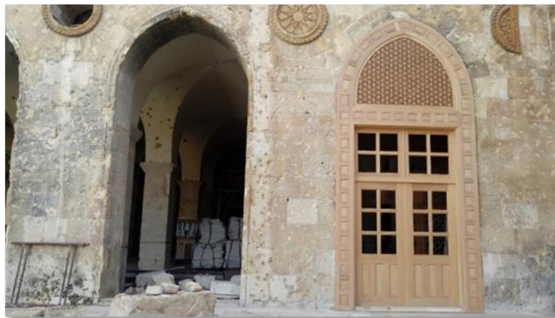
The manufacture and installation of the wooden works according to historical references of the finest types of wood and insulating paints
