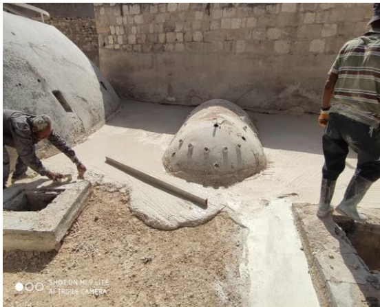
Implementing a moisture isolation layer to the roof
