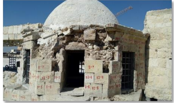
The stone dome of the Maqam was restored which was severely damaged by shells
