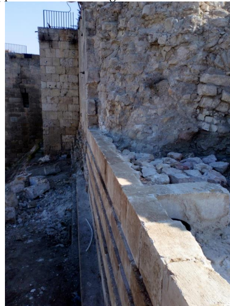
During the restoration works at the Northern wall
