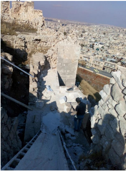
During the restoration works at the Eastern wall
