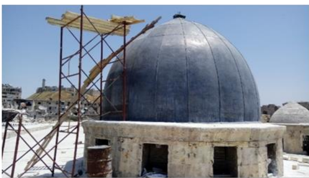
Restoration the damage domes in the courtyard of the mosque
