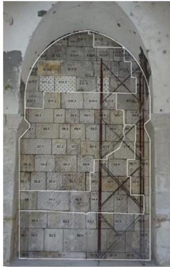
The restoration work in the Qibla in the mosque's includes documenting, dismantling, reconstructing and treating walls and columns, including cleaning and treating holes, filling mortar, and stone hammering.
