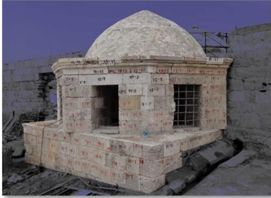
The stone dome of the Maqam was restored which was severely damaged by shells
