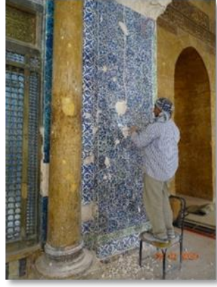
Maintenance and restoration of the shrine of the Prophet Zakaria included the manufacture of missing Qashani tiles for its internal and external facades and the maintenance of the old copper frames.
