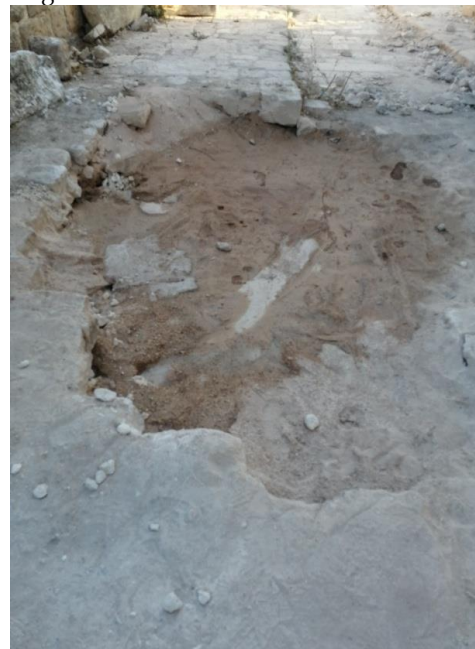
After filling the tunnels by soil and small stones
