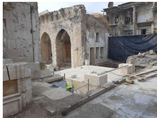
Rebuilding of the base of the minaret
