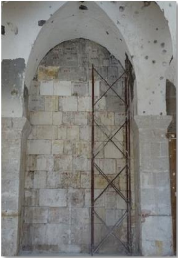
The restoration work in the Qibla in the mosque's includes documenting, dismantling, reconstructing and treating walls and columns, including cleaning and treating holes, filling mortar, and stone hammering.
