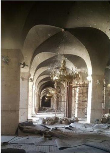
Peel and remove the damaged and burnt painting mortar and implement a new painting lime mortar in the walls and the roof of the Riwaq
