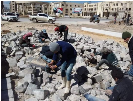
Above photo: Rehabilitating project in in Al Mutanabbi Street.
