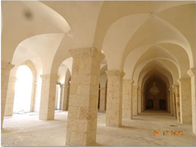
Peel and remove the damaged and burnt painting mortar and implement a new painting lime mortar in the walls and the roof of the Riwaq
