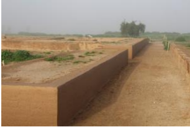
Figure 43. Mud-straw coating of architectural remains of Apadana
