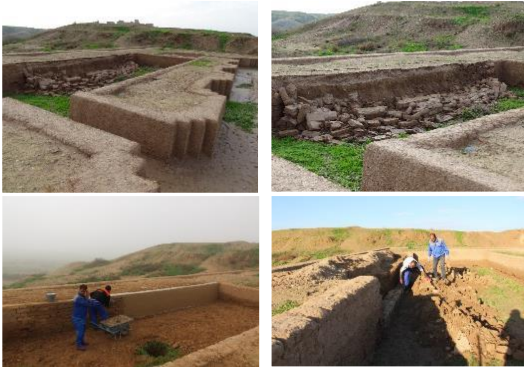
Figure ۴۸. Local restoration of eastern gate of Apadana Palace
