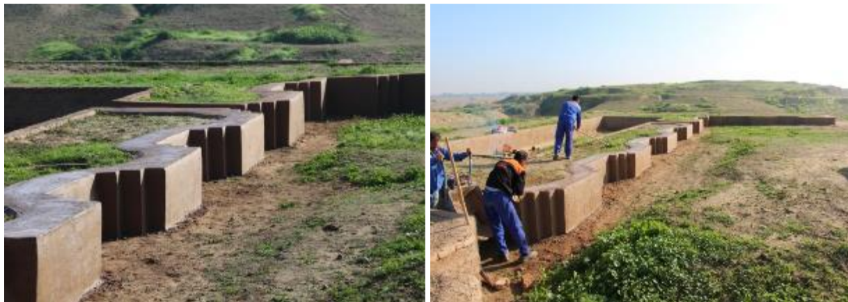
Figure 42. Mud-straw coating of remains of the eastern gate of Apadana
