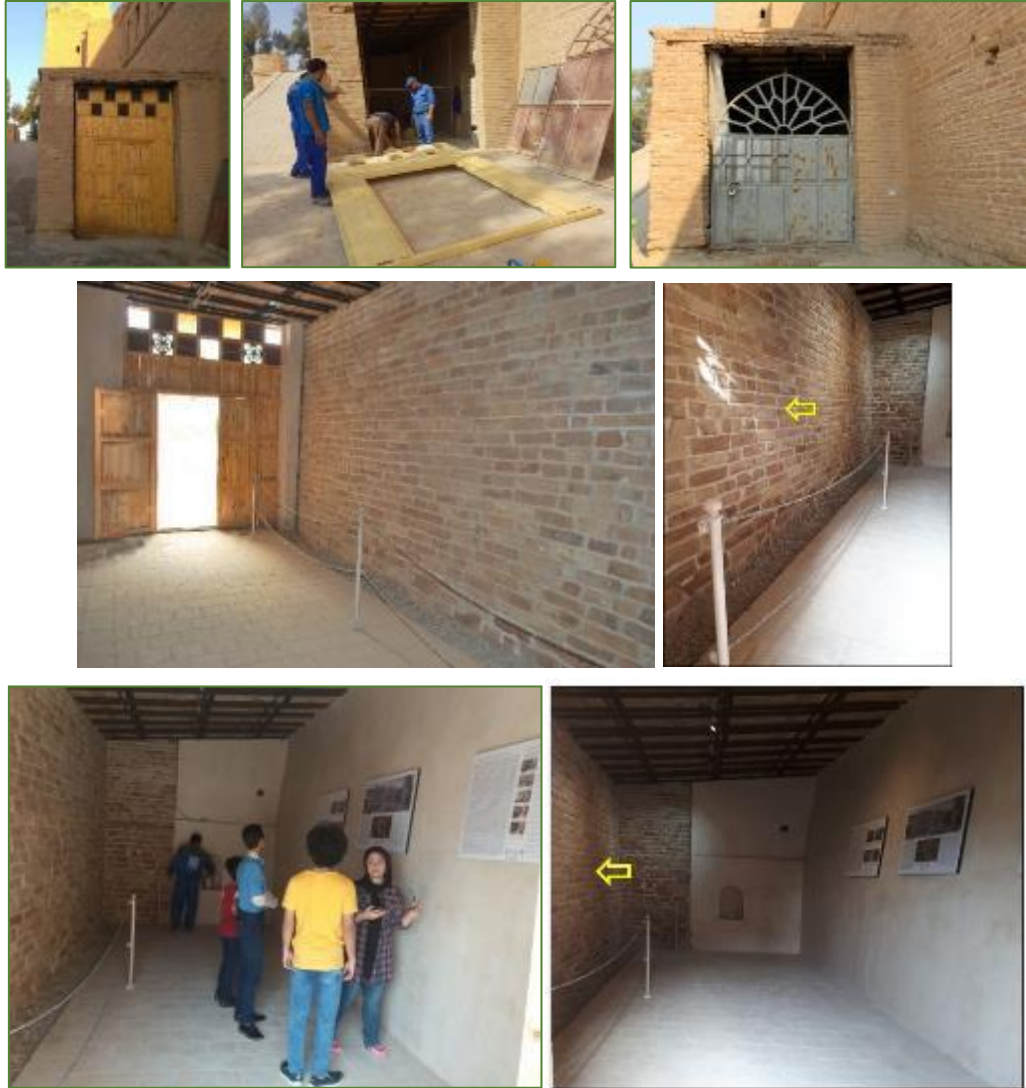
Figure ٥٢. Current condition of Girshman Garage after restoration
