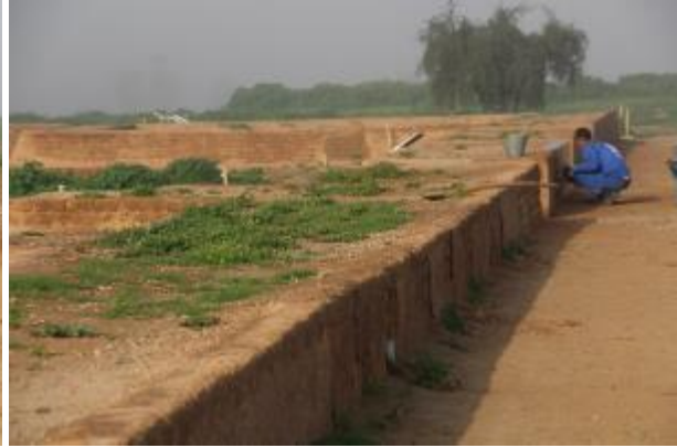
Figure 43. Mud-straw coating of architectural remains of Apadana
