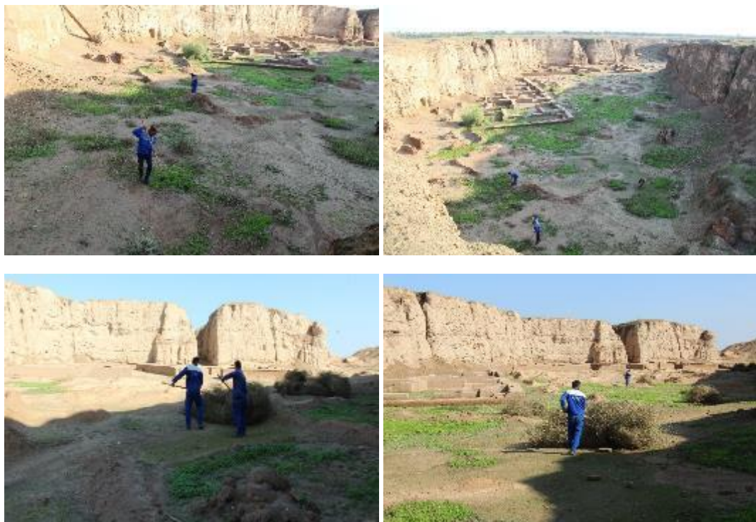
Figure 39. Removing vegetation within the large trench of Shahi town (fifteenth town)
