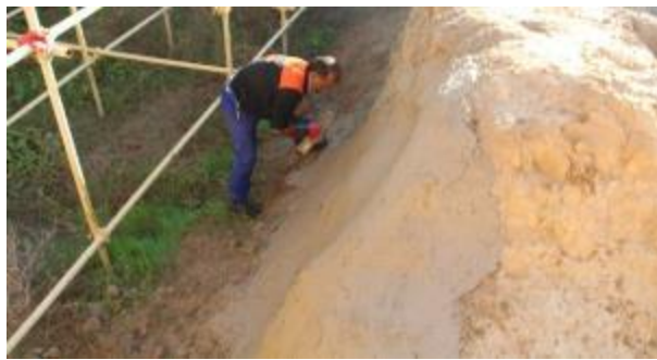
Figure 41. Mud-straw coating of remains in adobe-made pathway between Apadana Palace and Hadish
