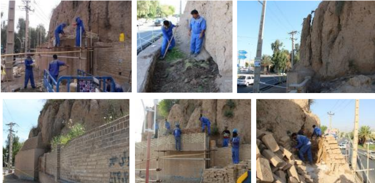
Figure 41 . Protective-restoration Measures on the northwestern tower of Apadana Royal Palace
