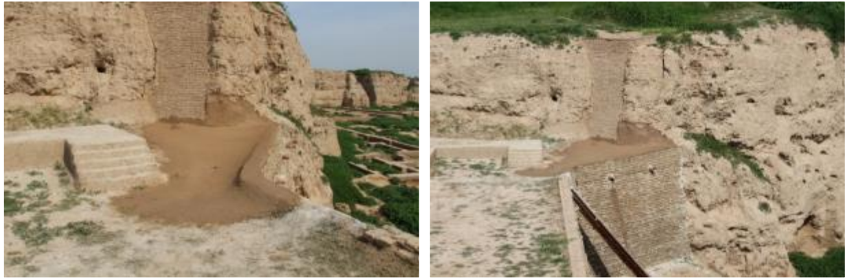
Figure 47. Restoration of water-washed edges of large trench of Shahi City (Fifteenth City)
