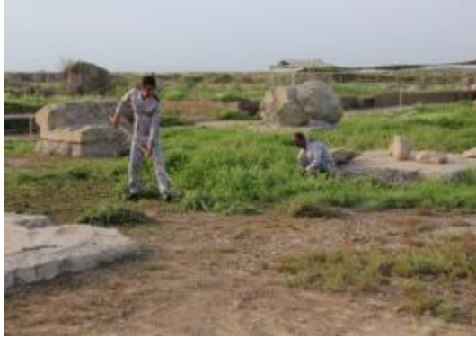
Figure 36. Removing Vegetation of the columned-hall of Apadana palace
