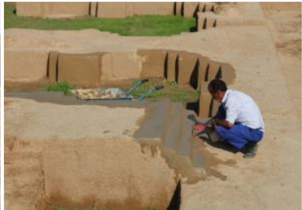
Figure 44. Mud-straw coating of architectural remains of Shavoor Palace
