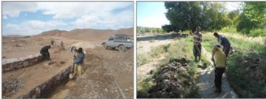
Figure 31. Dredging and modification of sides of Baladeh stream in adjacency of Baghestan Village (right); dredging Zaneh spring in initial water flowing section of Baladeh (2018, left)
