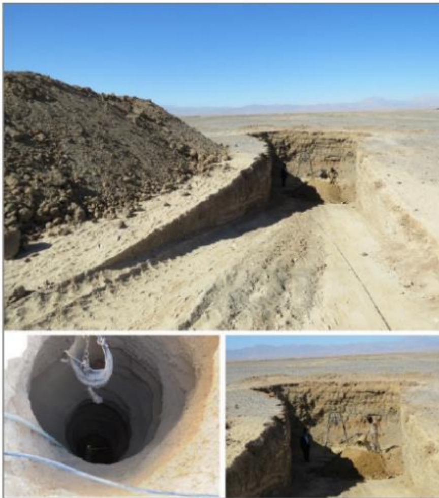
Figure 22. Dredging parts of Gonabad Qanat (2018)
