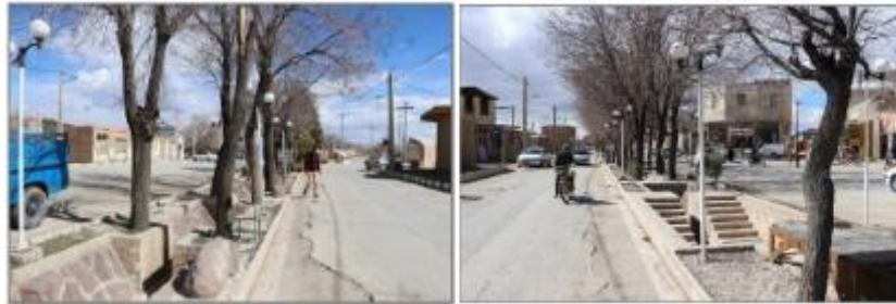
Figure 36. Cleaning the adjacent area of Qanat Mazhar (right) and removing improper furniture in the route leading to the Qanat (right, 2017)
