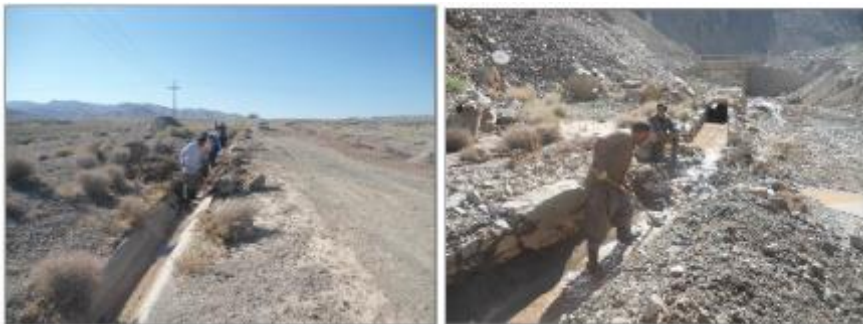
Figure 32. Dredging and removing flood debris in Shoqad Karriz (right) and dredging the streams of Shashtoo Karriz (left, 2019)
