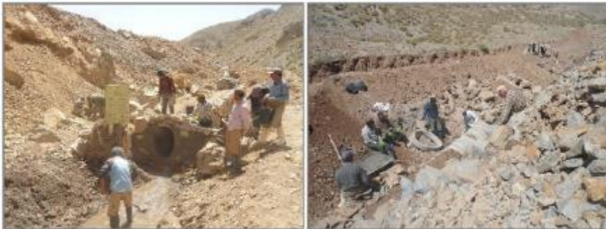
Figure 30. Restoration and construction of different parts of Shoqad Karriz (2019)
