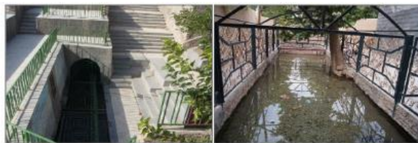
Figure 40. Restoration of Qanat outlet for optimal use of water (2018)
