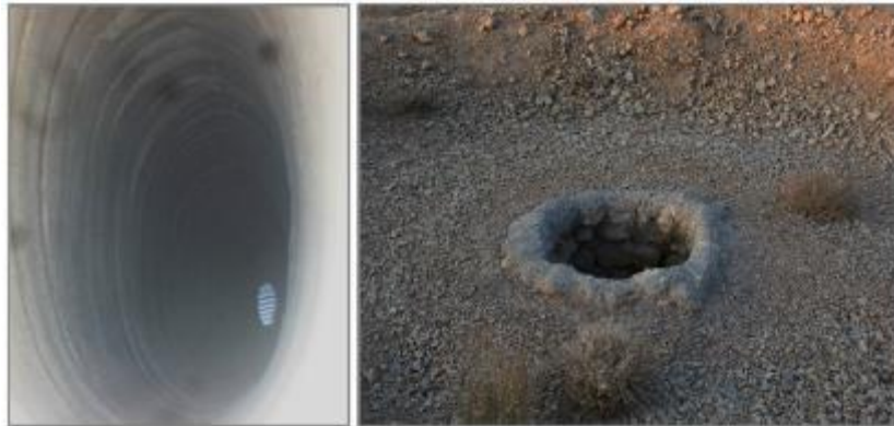
Figure 39. Restoration of well opening (right), reorganization of well shaft at entrance and exit of the site (2018)
