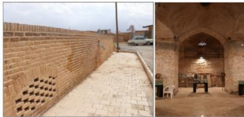
Figure 37. Cleaning internal space of water storage (right) and stone flooring of adjacent spaces of water storage (left, 2017)
