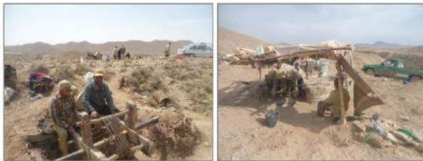
Figure 27. Dredging well shafts and Golavi Karriz Gallery (2018)
