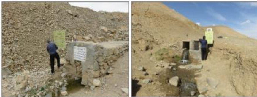
Figure 35. Installing a post with characteristics of Boreh Qanat in the area of Qanat outflowing gate (right) and installation of a post with characteristics of Shoqad Karriz at vicinity of Qanat outlet (left, 2019)
