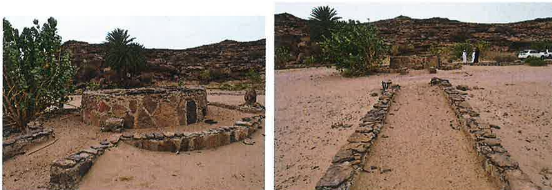
Concrete additions around the wells, to be removed on advice.
