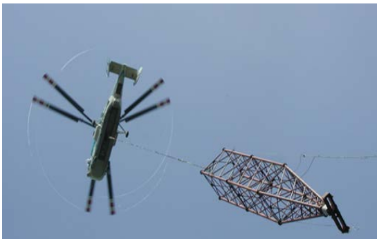
Figure 10: Helicopter carrying a tower during construction
