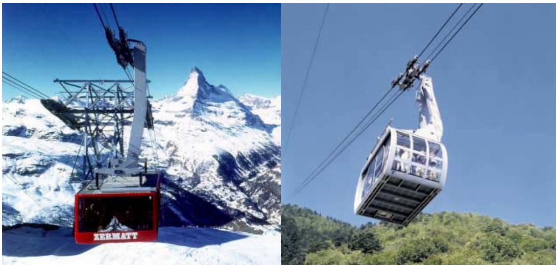
Figure 2: Cabins of aerial tramway system
