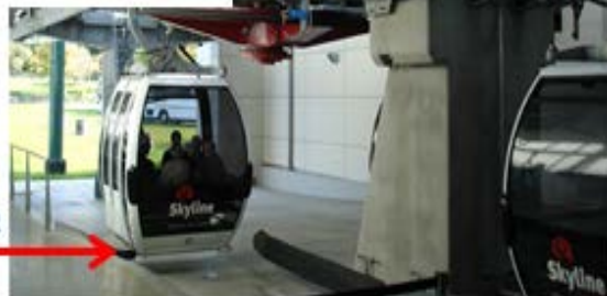
Fig. 1: station steel structure
