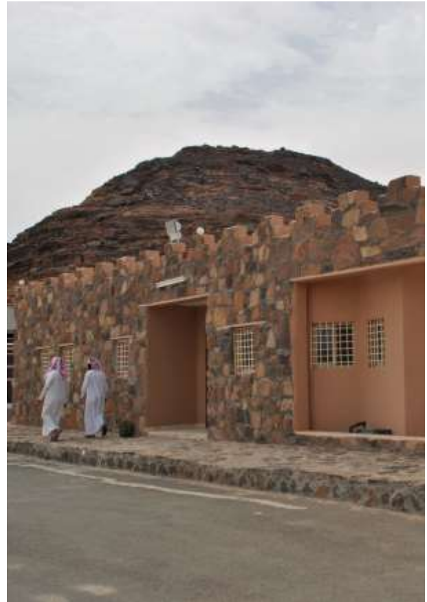
Figure 18. The existing Visitor Centre at Hima.
