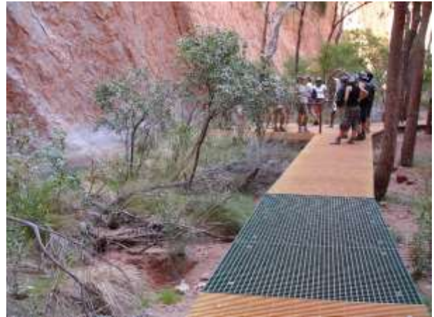
Figure 5.1 Raised walkways, like this example in Uluru WHS in Australia, can be used to keep visitors at a distance from rock surfaces, as well as improve access across a site
