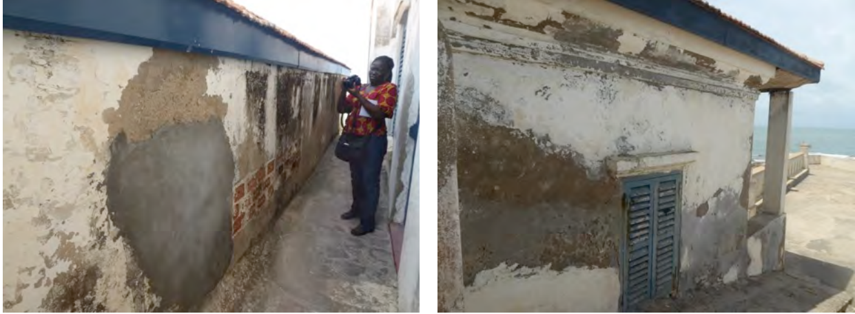
Figs. 23, 24 – Interventions with cement plaster instead of lime plaster at Cape Coast Castle
