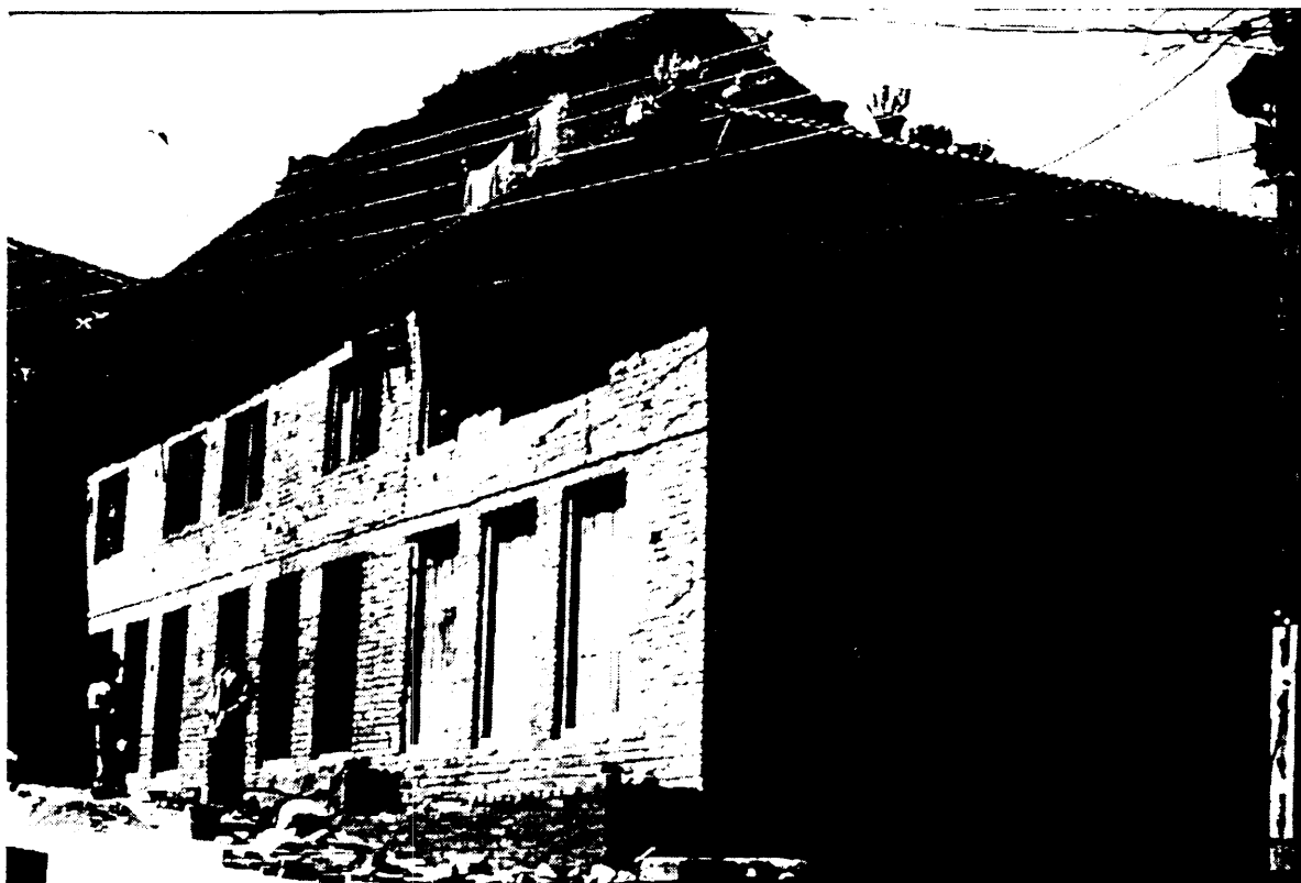
III. Changu 3. This illustration shows the illegal extension of the traditional house of Mr Ratna Bir Shrestha at Changu Narayan MZ. This extension can be corrected to conform to existing bylaws by adding a pitched roof (See Ch. 9 ICOMOS state of conservation, village of Changu Narayan). (c DM)
