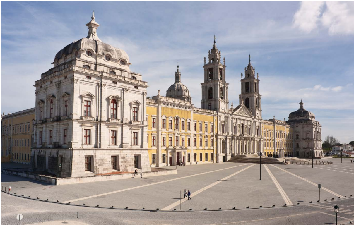
Main façade (east side)
