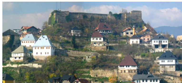
Figure 18. Reconstructed houses in the historic core of Jajce. © Commission to Preserve National Monuments of Bosnia and Herzegovina
