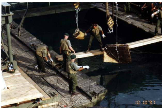
Figure 11. Collecting fragments of the Old Bridge in Mostar from the Neretva River in 1997. © Sulejman Demirović
