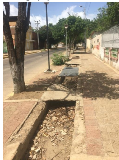
Photography 86: La Vela. Missing grids in the main street of the WH area
